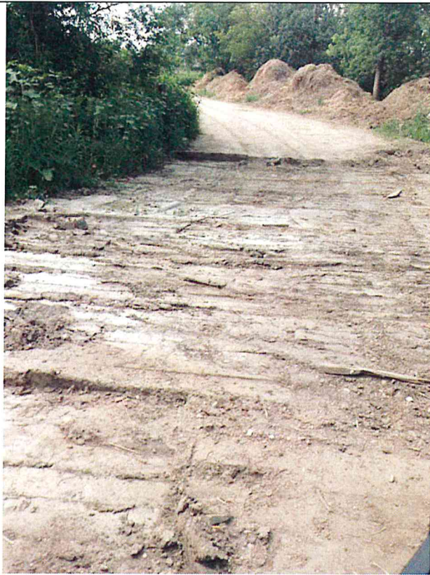
Photo 3: Adjacent to pole 68, showing rutting from recently removed construction matting within a wetland. This area will require further restoration.
