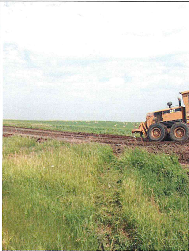
Photo 7: Road restoration activities as observed adjacent to Pole 31.
