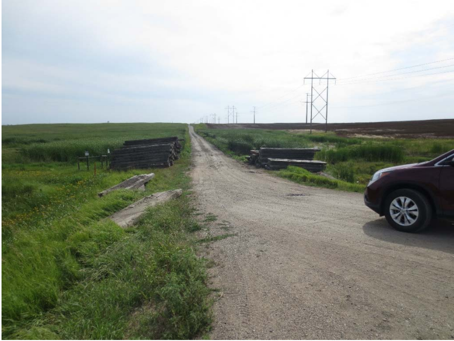
Photo 3: Pole 256 showing construction matting, looking east.
