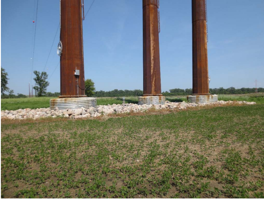
Photo 1: Pole 69 base, looking east across the Missouri River.
