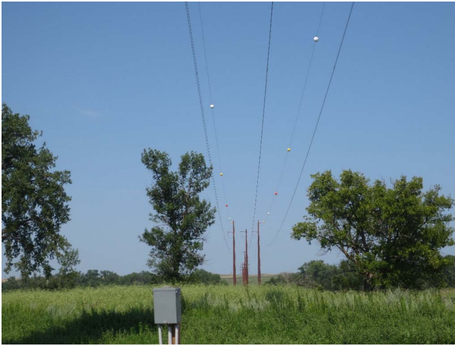
Photo 2: Pole 70, looking east across Missouri River.
