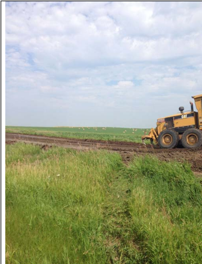
Photo 7: Road restoration activities as observed adjacent to Pole 31.
