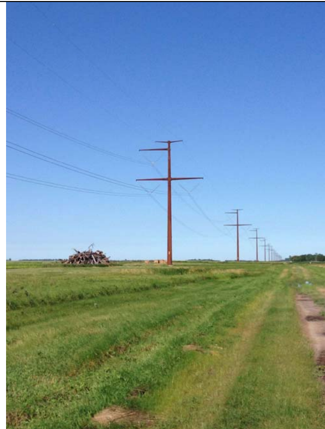
Photo 4: Pole 552, showing tree clearing areas and remnant debris.
