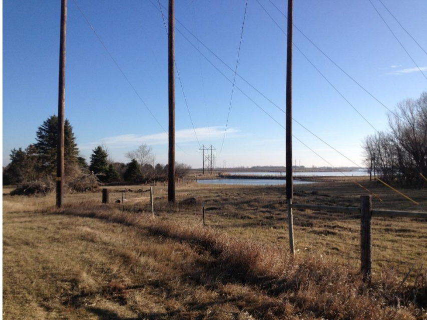
Photo 1. Direction: East. View of the first transmission structure installed for the reroute just east of 130 th Ave. SE in Section 14, Township 130 North, Range 56 West ( Figure 1 ).
