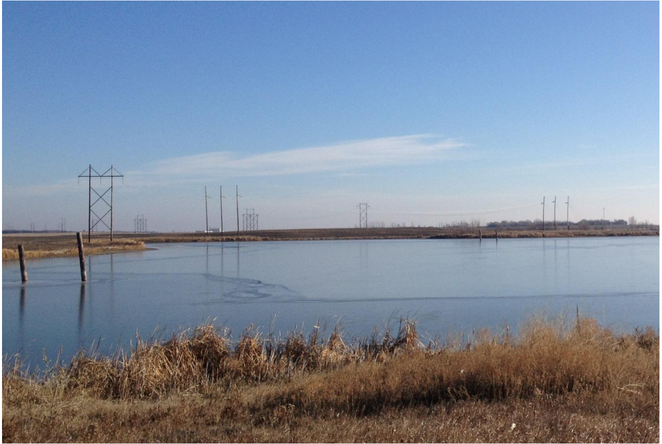
Photo 3. Direction: Northwest. View across Fiala Lake towards the rerouted transmission line. Two tangents were used to route the transmission line; both were located nearby the Lake, but only one was within close proximity, and it had riprap installed to prevent erosion and to protect the structure. No erosion or sedimentation was observed to the Lake. By request, the landowner will remove the old poles when they float to the surface (seen to the left and across the lake to the right).
