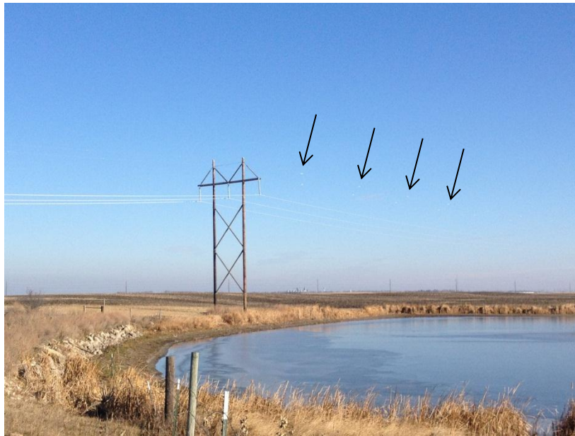
Photo 2. Direction: Northeast. View of the transmission line showing bird diverters along the line, which are faintly visible (indicated by black arrows).
