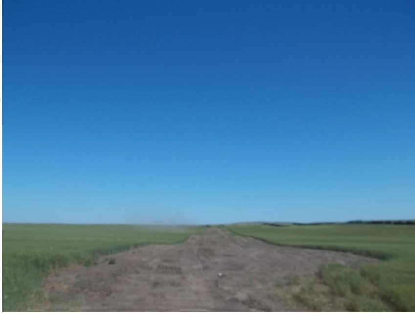
Photo 99. Direction: North. This photo shows the right-of-way for the Bridger Pipeline. At the time of our site visit the right-of-way needed final restoration.
