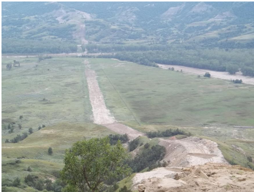
Photo 68. Direction: South. This photo shows the right-of-way for the Bridger Pipeline. At the time of our site visit the area shown needed slope contour fixed and final restoration.
