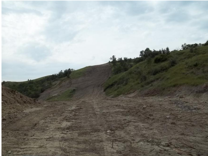
Photo 65. Direction: South. This photo shows the right-of-way for the Bridger Pipeline. At the time of our site visit the right-of-way needed final restoration.
