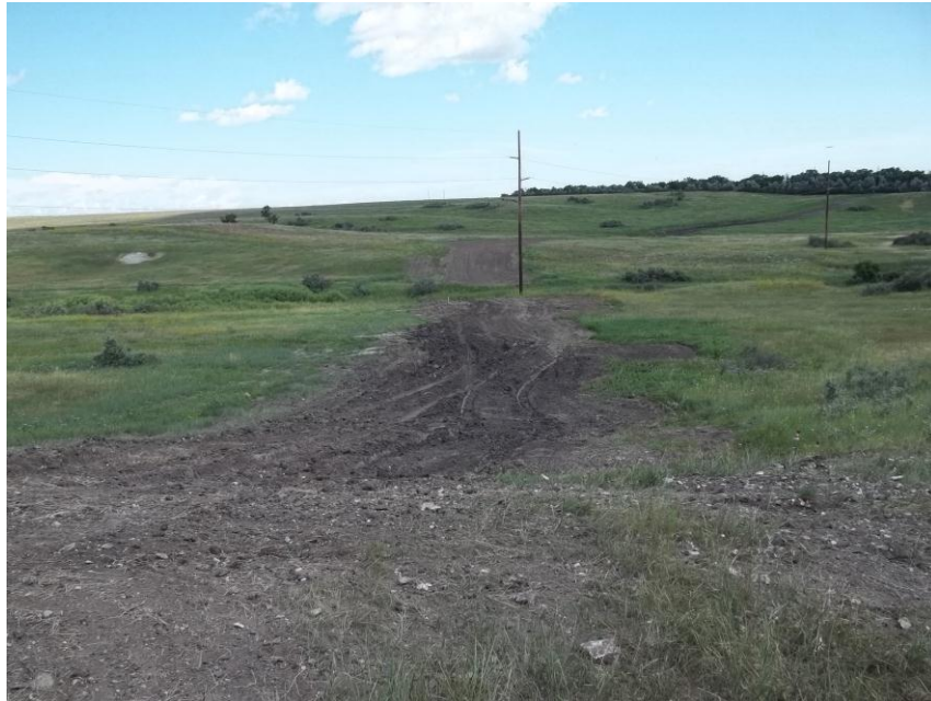
Photo 37. Direction: North. This photo shows the right-of-way for the Bridger Pipeline. At the time of our site visit the right-of-way needed final restoration.
