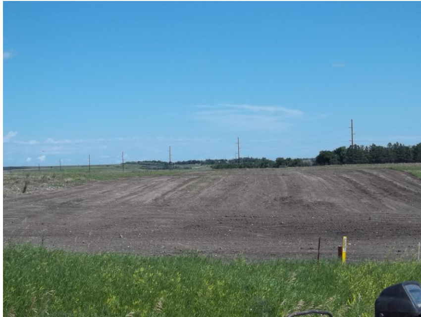
Photo 33. Direction: North. This photo shows the right-of-way for the Bridger Pipeline. At the time of our site visit the right-of-way needed final restoration.
