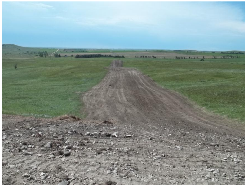
Photo 26. Direction: South. This photo shows the right-of-way for the Bridger Pipeline. At the time of our site visit the right-of-way needed final restoration.
