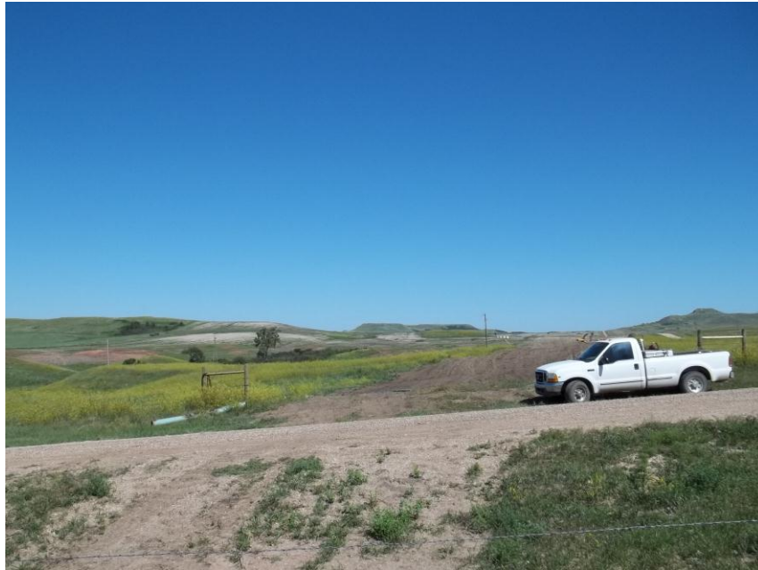
Photo 111. Direction: North. This photo shows the right-of-way for the Bridger Pipeline. At the time of our site visit the right-of-way needed final restoration.
