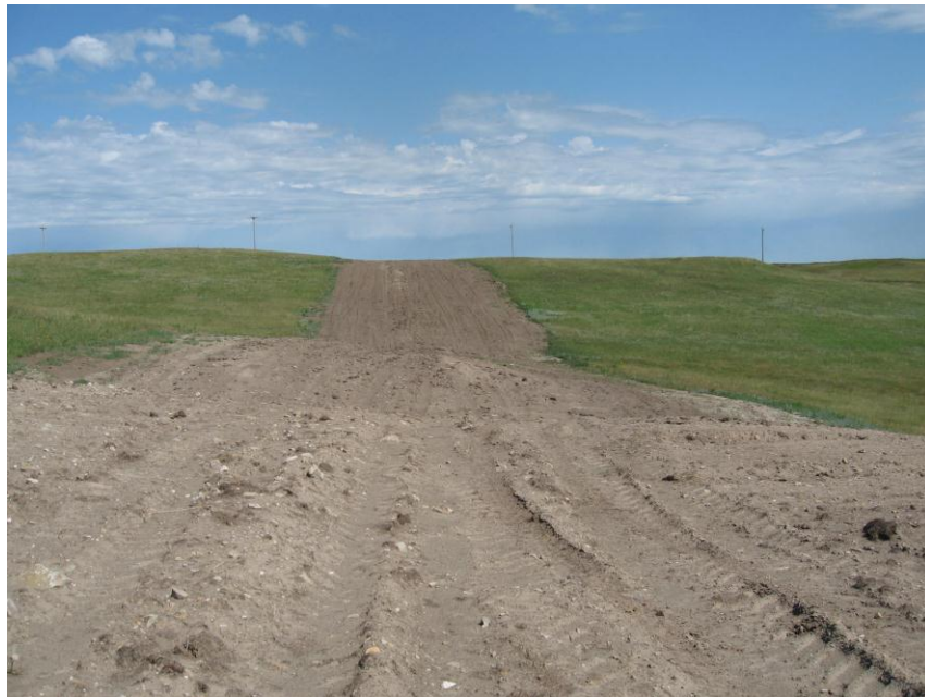
Photo 6. Direction: North. This photo shows the right-of-way for the Bridger Pipeline. At the time of our site visit the right-of-way needed final restoration.
