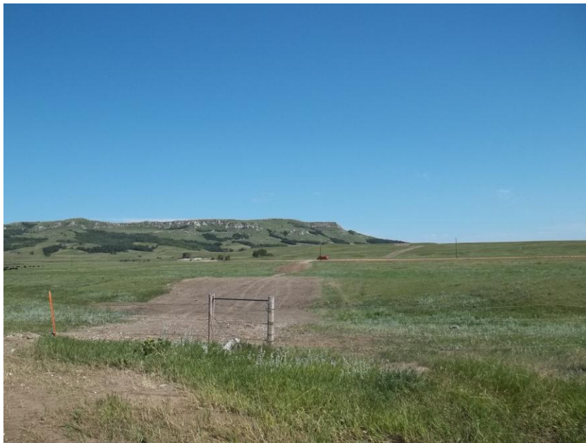
Photo 24. Direction: North. This photo shows the right-of-way for the Bridger Pipeline. At the time of our site visit the right-of-way needed final restoration.
