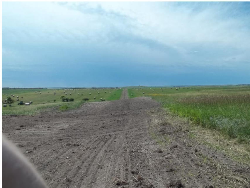
Photo 22. Direction: South. This photo shows the right-of-way for the Bridger Pipeline. At the time of our site visit the right-of-way needed final restoration.
