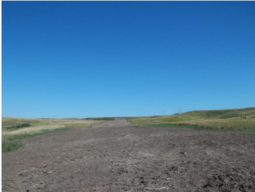
Photo 93. Direction: North. This photo shows the right-of-way for the Bridger Pipeline. At the time of our site visit the right-of-way needed final restoration.
