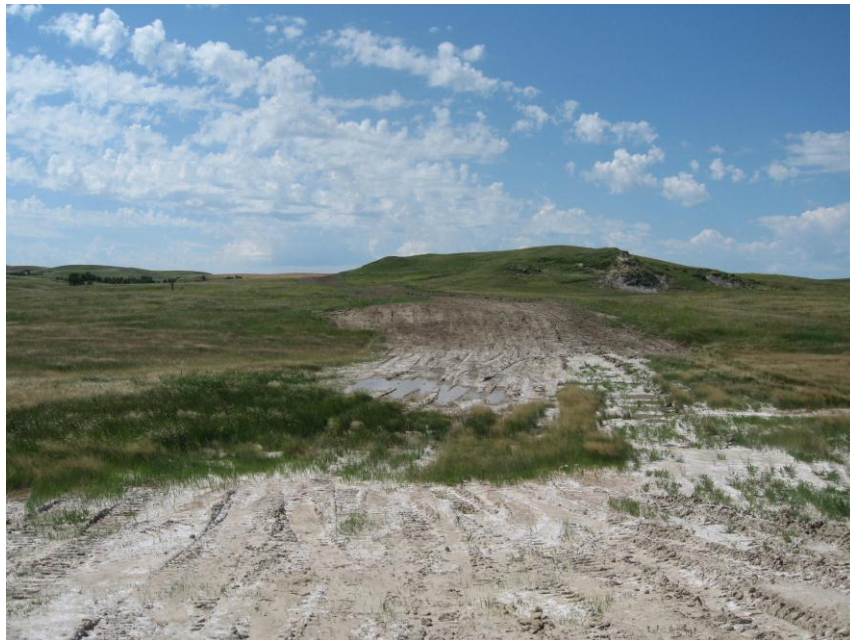
Photo 8. Direction: North. This photo shows the right-of-way for the Bridger Pipeline. At the time of our site visit the right-of-way needed final restoration.
