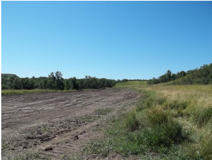
Photo 102. Direction: South. This photo shows the right-of-way for the Bridger Pipeline. At the time of our site visit the right-of-way needed final restoration.
