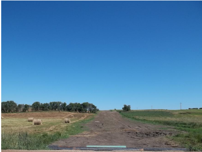
Photo 97. Direction: North. This photo shows the right-of-way for the Bridger Pipeline. At the time of our site visit the right-of-way needed final restoration.
