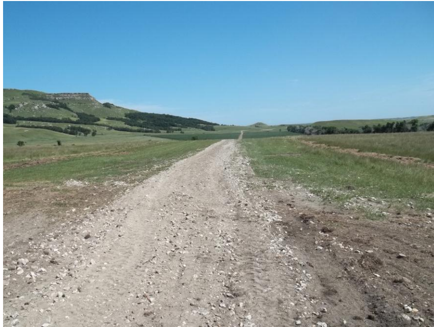
Photo 27. Direction: North. This photo shows the right-of-way for the Bridger Pipeline. At the time of our site visit the right-of-way needed final restoration.
