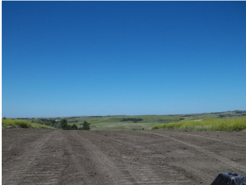
Photo 129. Direction: North. This photo shows the right-of-way for the Bridger Pipeline. At the time of our site visit the right-of-way needed final restoration.
