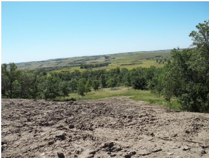
Photo 120. Direction: South. This photo shows the right-of-way for the Bridger Pipeline. At the time of our site visit the right-of-way needed final restoration.
