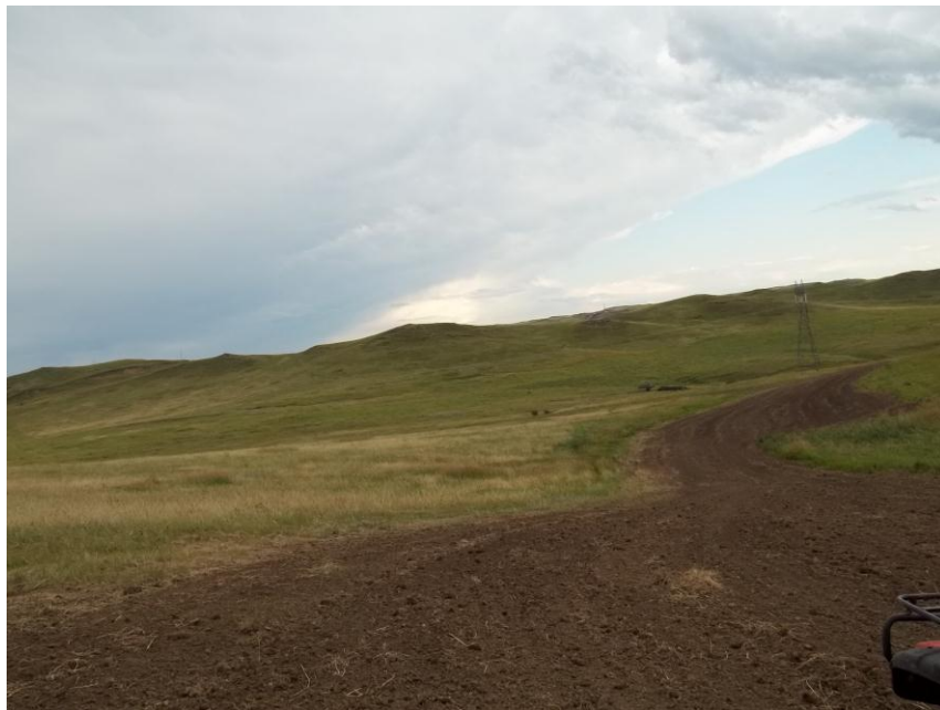
Photo 12. Direction: South. This photo shows the right-of-way for the Bridger Pipeline. At the time of our site visit the right-of-way needed final restoration.
