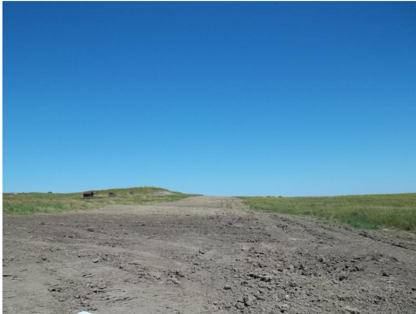
Photo 119. Direction: North. This photo shows the right-of-way for the Bridger Pipeline. At the time of our site visit the right-of-way needed final restoration.
