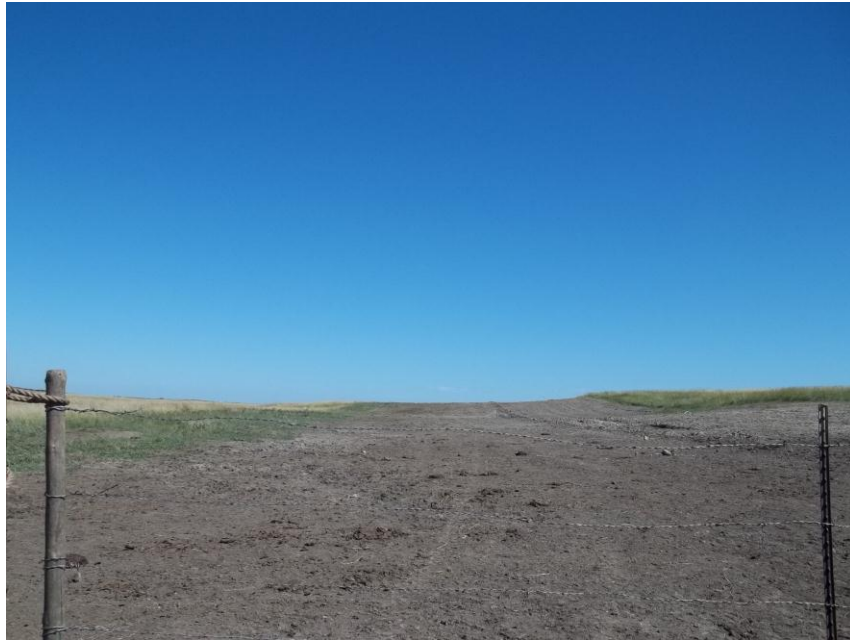
Photo 91. Direction: North. This photo shows the right-of-way for the Bridger Pipeline. At the time of our site visit the right-of-way needed final restoration.
