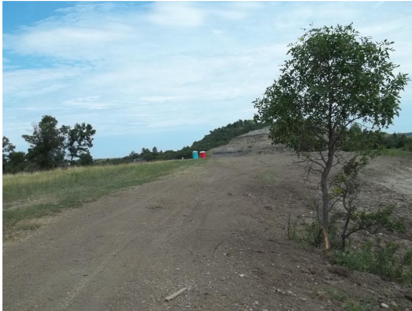
Photo 75. Direction: South. This photo shows the right-of-way for the Bridger Pipeline. At the time of our site visit the right-of-way needed final restoration.
