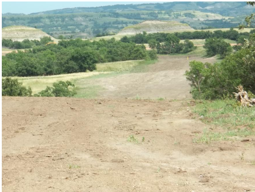
Photo 72. Direction: North. This photo shows the right-of-way for the Bridger Pipeline. At the time of our site visit the right-of-way needed final restoration.
