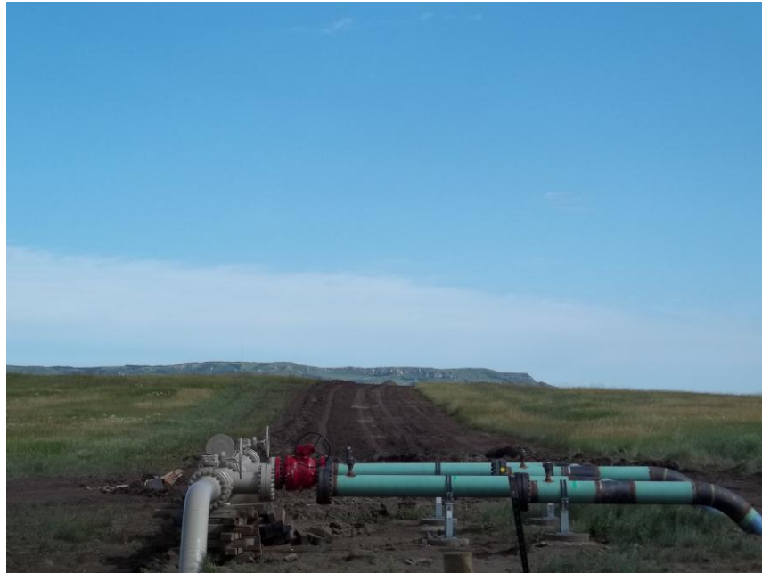
Photo 17. Direction: North. This photo shows the right-of-way for the Bridger Pipeline. At the time of our site visit the right-of-way needed final restoration.
