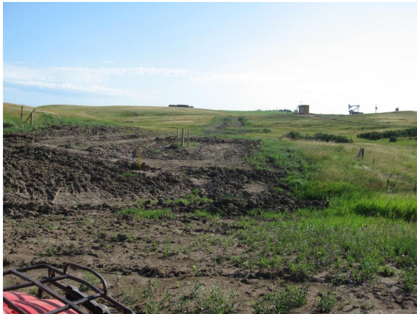
Photo 2. Direction: Northeast. This photo shows the right-of-way for the Bridger Pipeline. At the time of our site visit the right-of-way had wet soil conditions and needed final restoration.
