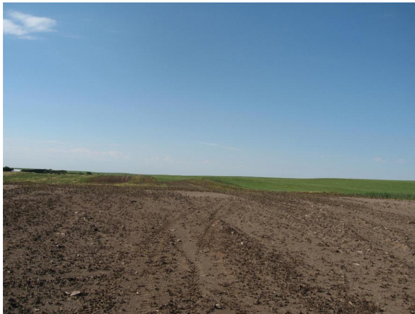
Photo 4. Direction: North. This photo shows the right-of-way for the Bridger Pipeline. At the time of our site visit the area shown had wet soil conditions and needed final restoration.
