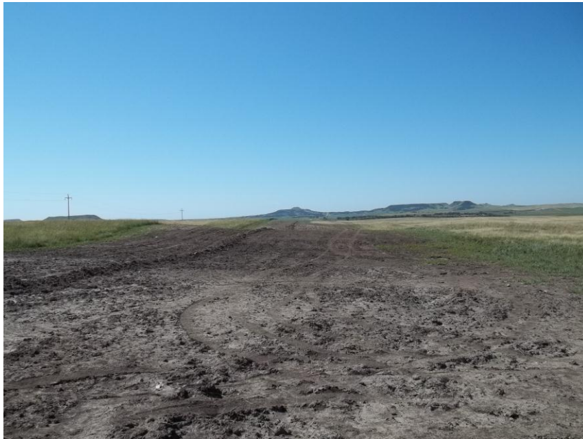
Photo 90. Direction: South. This photo shows the right-of-way for the Bridger Pipeline. At the time of our site visit the right-of-way needed final restoration.
