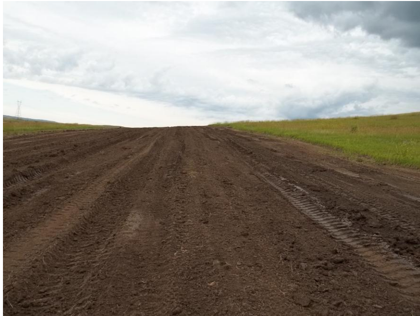
Photo 15. Direction: Northeast. This photo shows the right-of-way for the Bridger Pipeline. At the time of our site visit the right-of-way needed final restoration.
