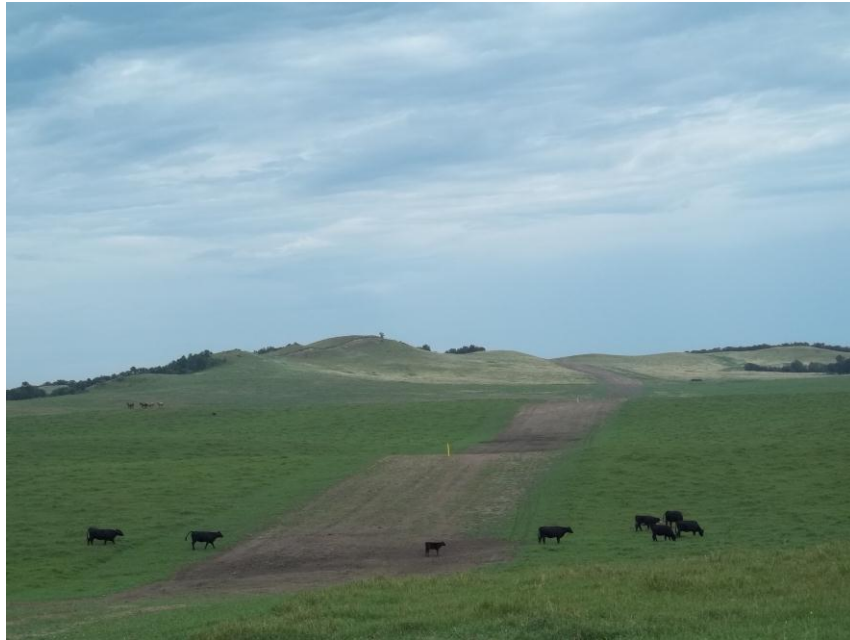
Photo 69. Direction: North. This photo shows the right-of-way for the Bridger Pipeline. At the time of our site visit the right-of-way needed final restoration.
