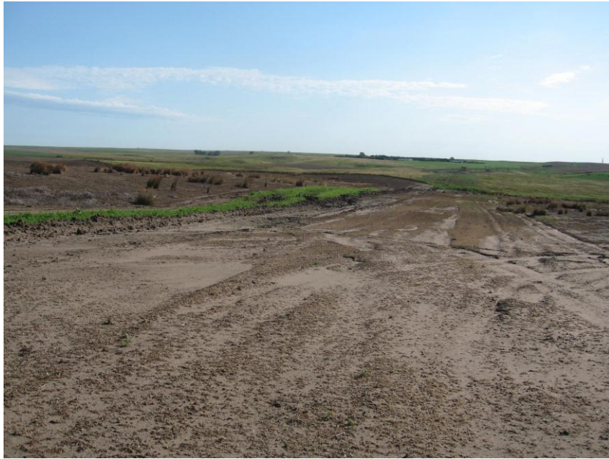
Photo 1. Direction: Northeast. This photo shows the right-of-way for the Bridger Pipeline. At the time of our site visit the right-of-way needed final restoration.
