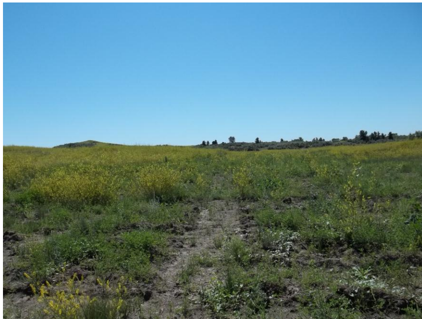
Photo 130. Direction: Southwest. This photo shows the right-of-way for the Bridger Pipeline. At the time of our site visit the right-of-way needed final restoration.
