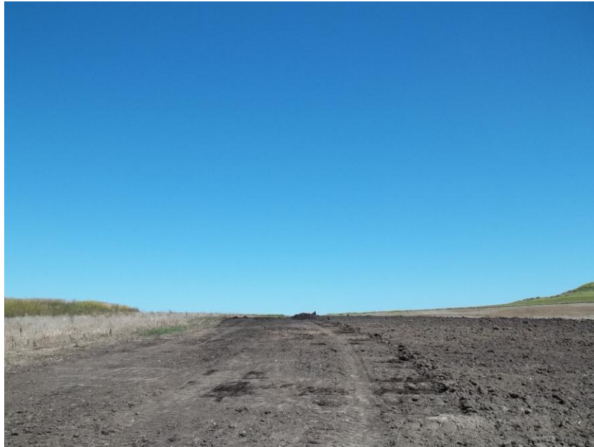
Photo 115. Direction: North. This photo shows the right-of-way for the Bridger Pipeline. At the time of our site visit the right-of-way needed final restoration.
