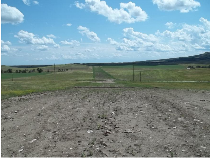
Photo 51. Direction: South. This photo shows the right-of-way for the Bridger Pipeline. At the time of our site visit the right-of-way needed final restoration.
