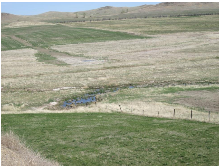
Photo 36. Direction: Northeast. Pipeline right-of-way where it was bored under the Little Knife River. No erosion or sedimentation to the waterbody was evident.
