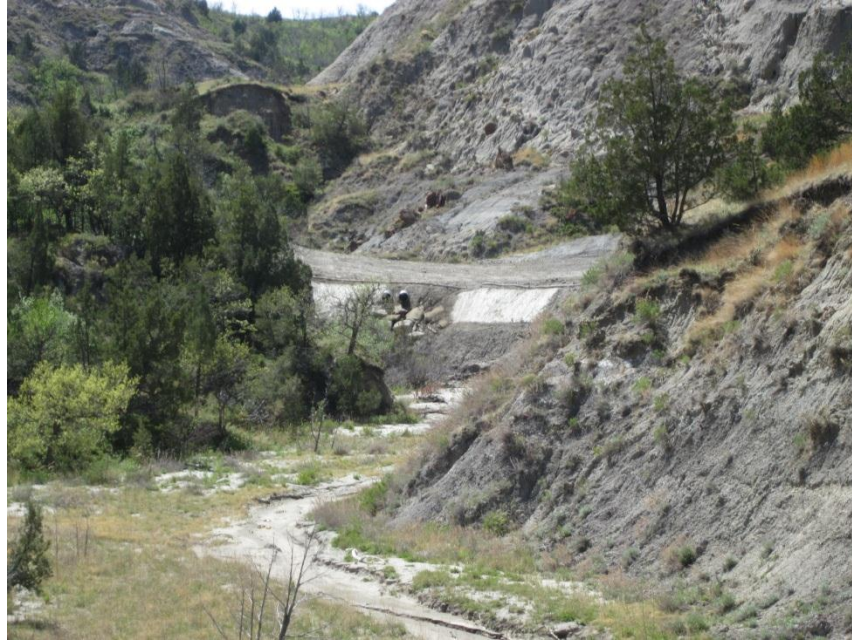
Photo 55. Direction: West. Photo shows an area where erosion had been a problem. Erosion was controlled by diverting water through culverts and laying down grass mats. It appeared these methods have been successful.
