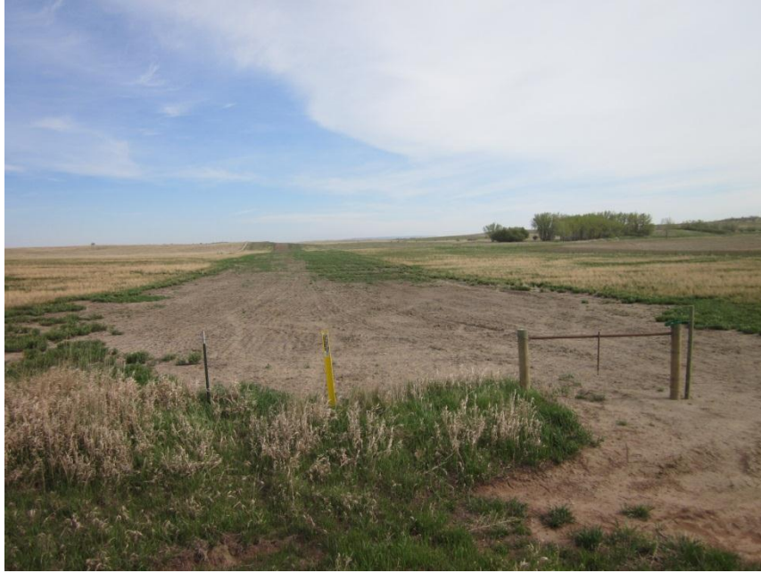
Photo 7. Direction: North. Pipeline right-of-way. Note repaired fence and posted signage.
