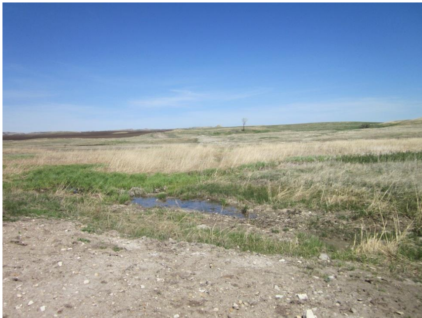
Photo 42. Direction: South. Photo shows an area where Bridger’s pipeline bored under a wetland. No erosion or sedimentation to the water body was evident. Some ponding was noted on the right-of-way.
