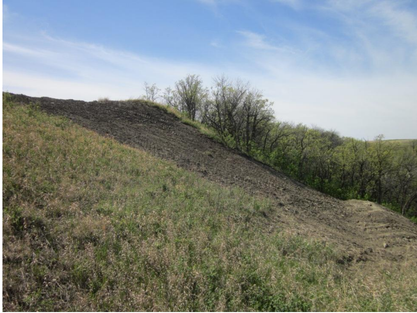
Photo 59. Direction: West. Note water bar and soil recontouring on the slope.
