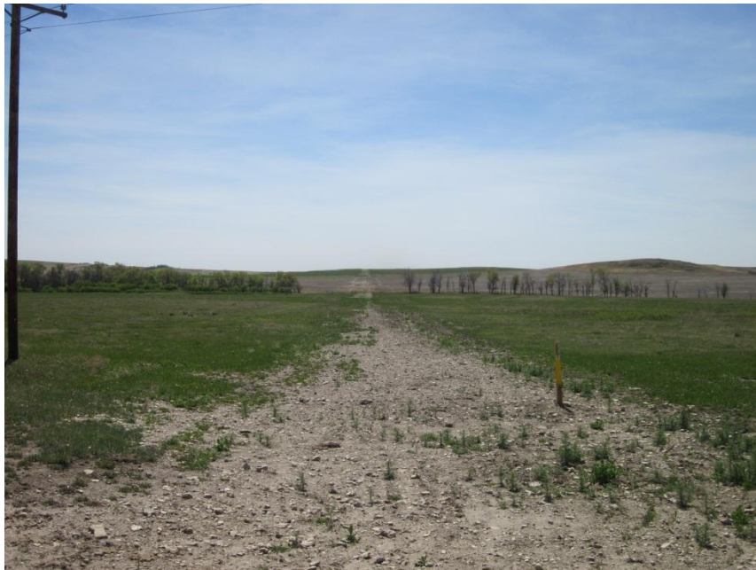
Photo 44. Direction: South. Photo shows the right-of-way of Bridger's pipeline in an area with rocky soils. Rocks had been picked prior to reseeding but it appeared some resurfaced.
