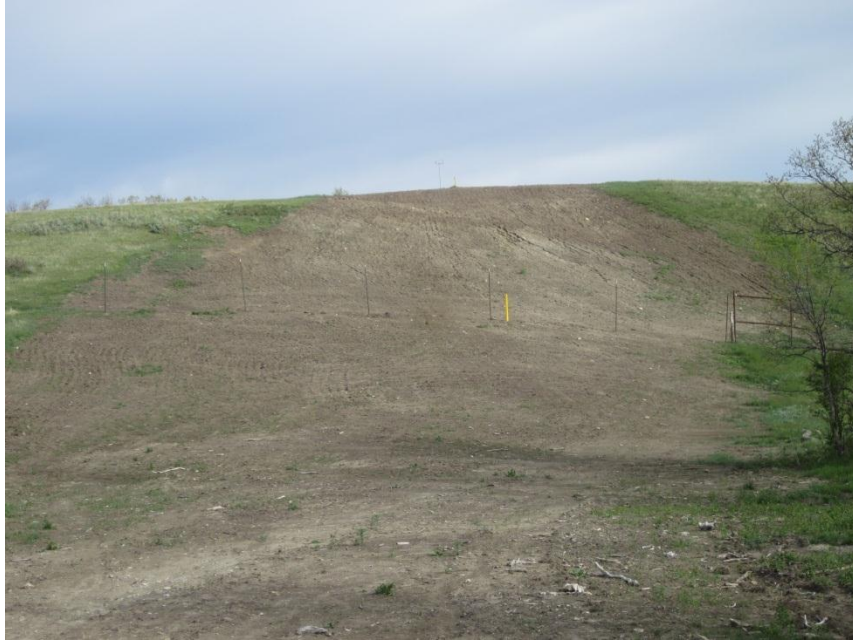
Photo 69. Direction: North. Pipeline right-of-way. Note buffalo fence that had been replaced.
