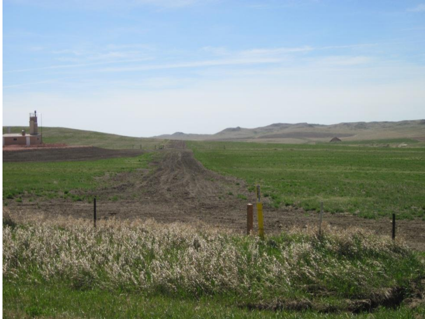
Photo 33. Direction: South. Pipeline right-of-way. Reseeding had occurred, but vegetation had yet to reclaim the disturbance.
