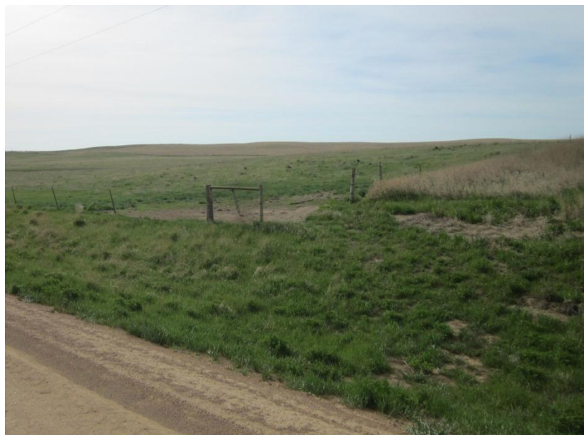
Photo 6. Direction: Southeast. An access road for Bridger's pipeline routed through the fenceline just below the dense grass in the upper right hand corner of the photo. Disturbance had been restored and almost completely reclaimed.
