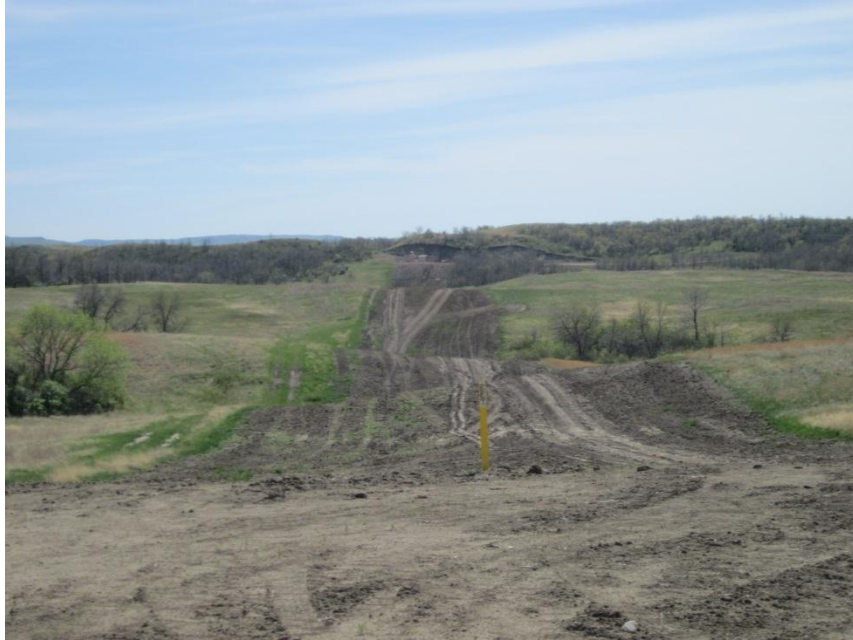
Photo 57. Direction: South. Pipeline right-of-way. Restoration and reseeded had occurred, but vegetation had yet to reclaim the area.
