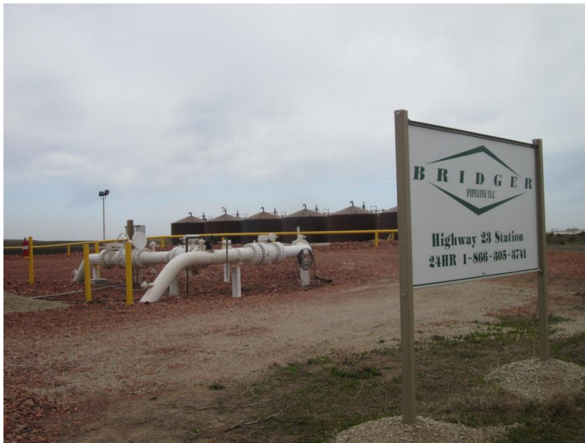
Photo 78. Direction: West. Station 23, the end of Bridger's pipeline.
