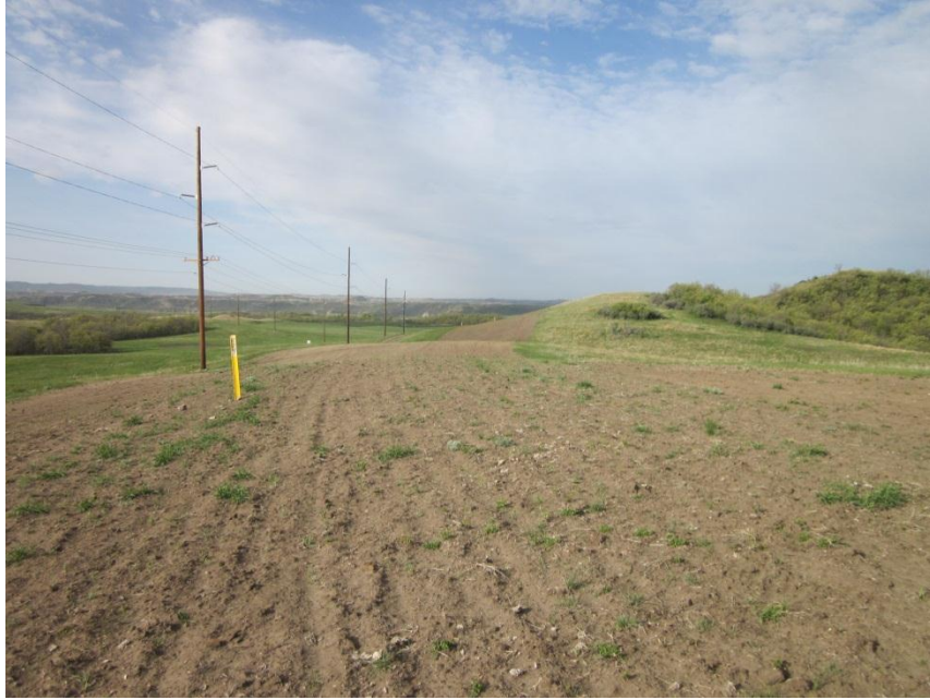
Photo 63. Direction: East. Pipeline right-of-way. Reseeding had occurred, but vegetation had yet to reclaim the disturbance.
