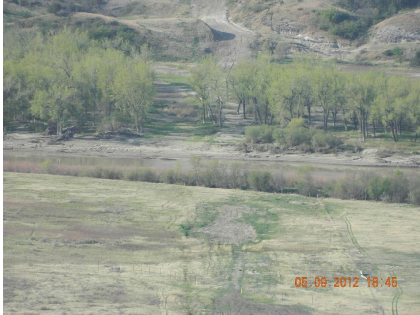
Photo 61. Direction: South. Photo shows where the right-of-way of Bridger’s pipeline bores under the Little Missouri River. No erosion or sedimentation was evident to the water body.
