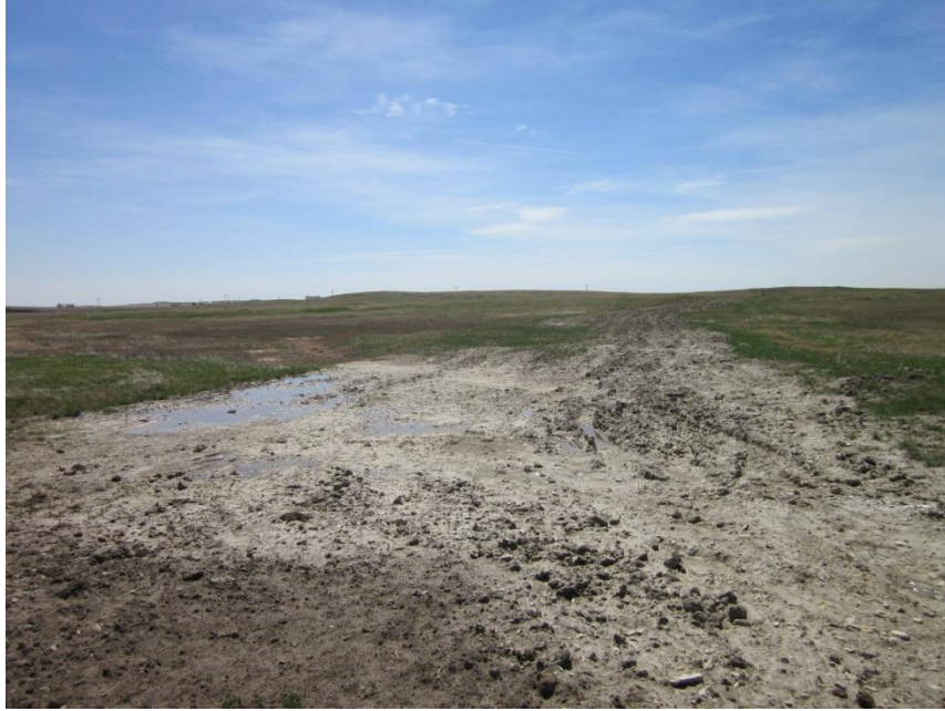
Photo 41. Direction: South. Photo shows the right-of-way of Bridger’s pipeline north of a wetland crossing. There was some ponding of water along the right-of-way.
