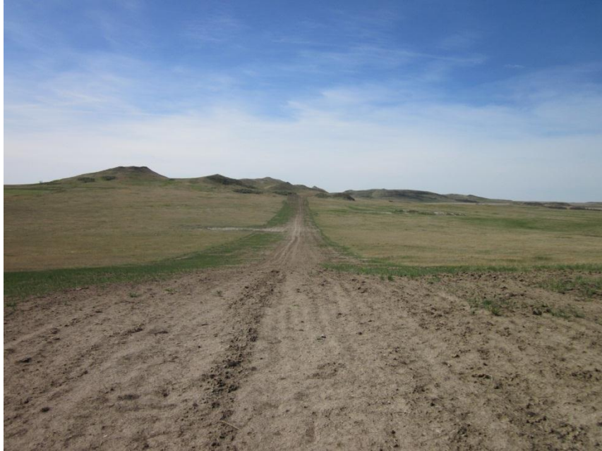
Photo 19. Direction: South. Pipeline right-of-way just north of Photo 18. Reseeding had occurred, but vegetation had yet to reclaim the disturbance.
