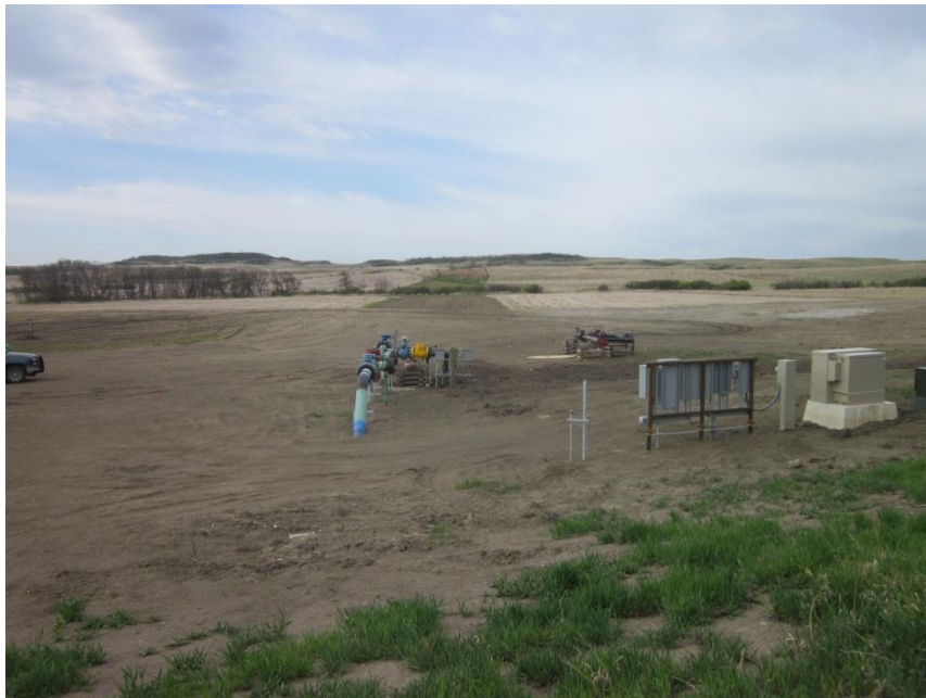
Photo 70. Direction: South. Photo shows the right-of-way of Bridger's pipeline 73 rd interconnect.
