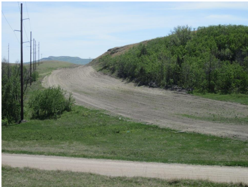
Photo 52. Direction: South. Pipeline right-of-way. Disturbance had been limited to 50ft where the pipeline routed through this wooded area.
