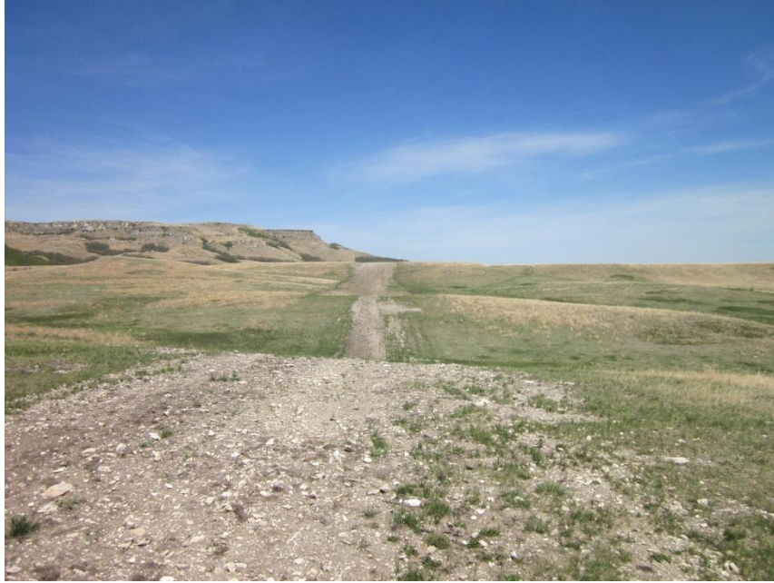
Photo 45. Direction: North. Photo shows the right-of-way of Bridger’s pipeline in an area with rocky soils. Rocks had been picked prior to reseeding but it appeared some resurfaced.
