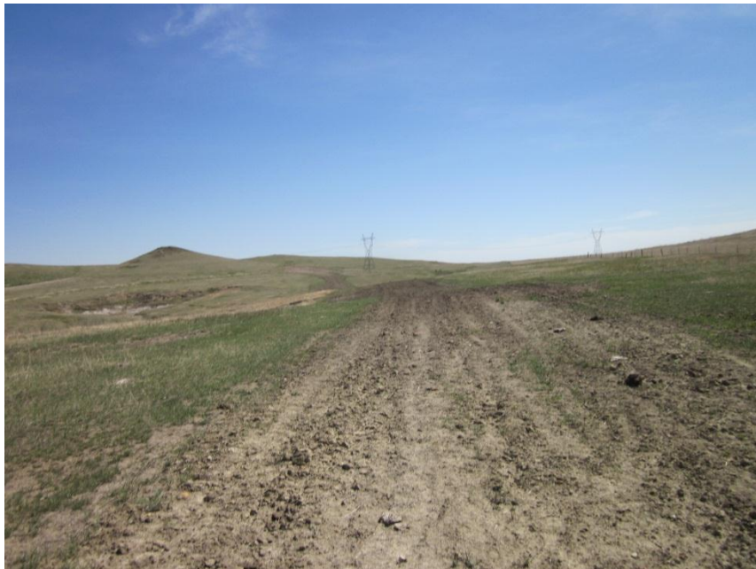
Photo 38. Direction: Northeast. Pipeline right-of-way. Reseeding had occurred, but vegetation had yet to reclaim the disturbance.
