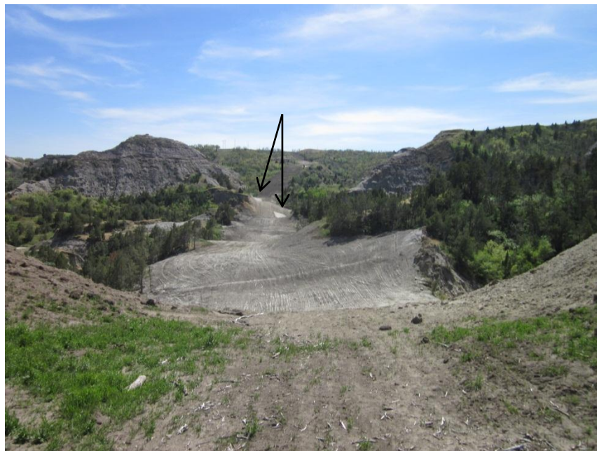
Photo 56. Direction: South. Pipeline right-of-way. Note grass mats in place to prevent erosion (indicated by arrows).
