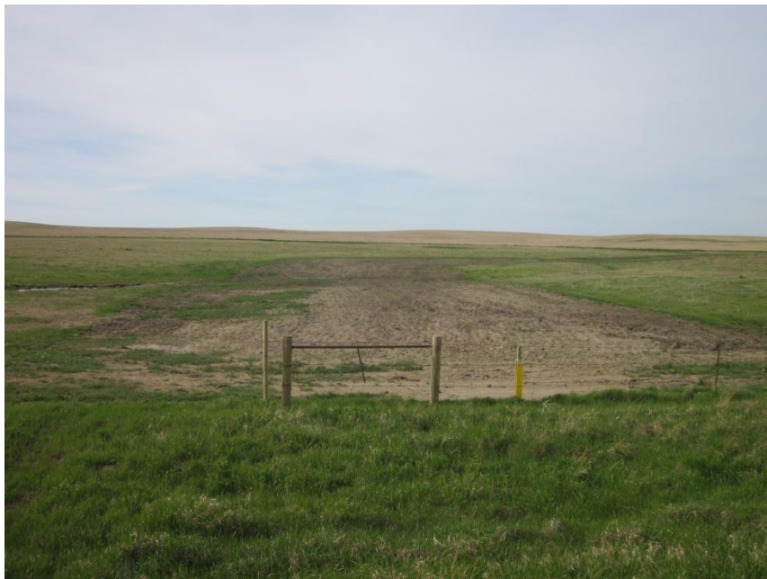
Photo 4. Direction: South. Pipeline right-of-way. Note repaired fence and signage where the pipeline crosses the fenceline.
