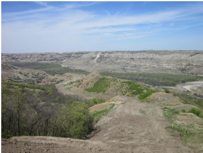
Photo 58. Direction: Northwest. Low soil cohesion caused major erosion problems. Soil was hauled in and water bars were installed. The slope appeared to be stabilized.
