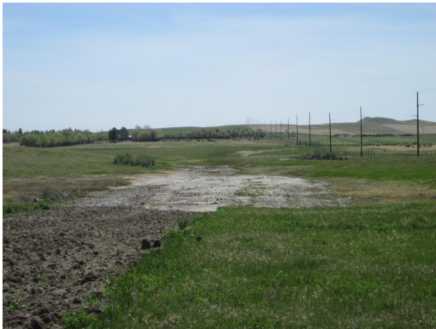
Photo 48. Direction: South. Pipeline right-of-way. This wet area had caused construction problems, but restoration appeared to have ameliorated any permanent impacts.
