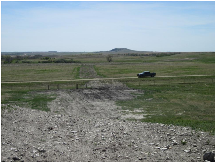
Photo 46. Direction: South. Photo shows the right-of-way of Bridger’s pipeline. Roadway was bored and in good condition.
