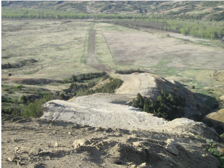
Photo 60. Direction: South. Photo shows the right-of-way of Bridger's pipeline north of the Little Missouri. Recontouring and water bars controlled erosion, but vegetation had yet to reclaim the slope.
