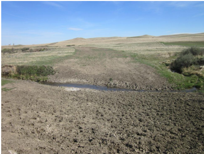
Photo 14. Direction: North. Photo shows Bridger's pipeline where it crosses Crooked Creek.
