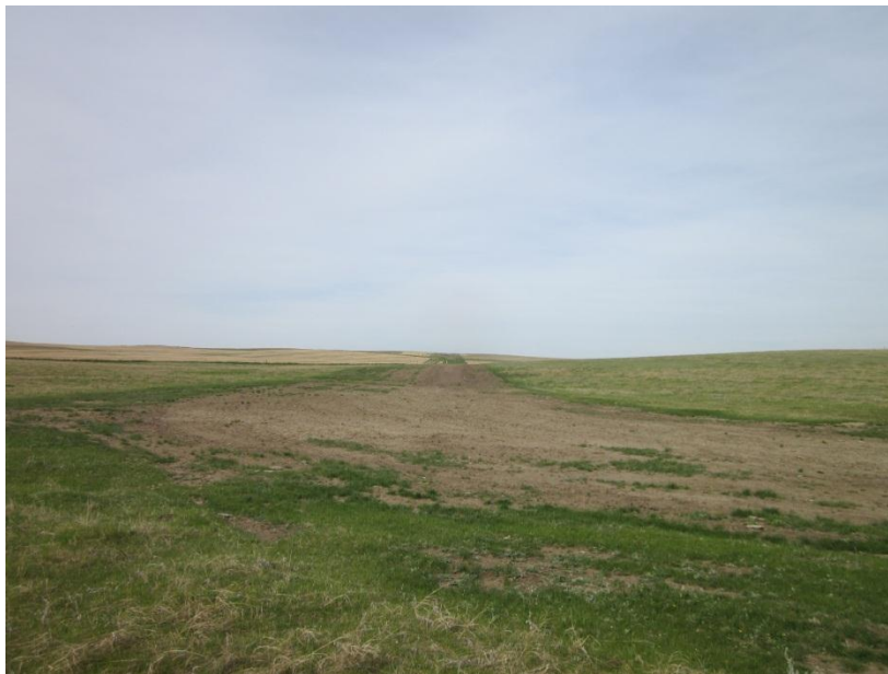
Photo 2. Direction: Southwest. Pipeline right-of-way. Reseeding had occurred, but vegetation had yet to reclaim the disturbance.
