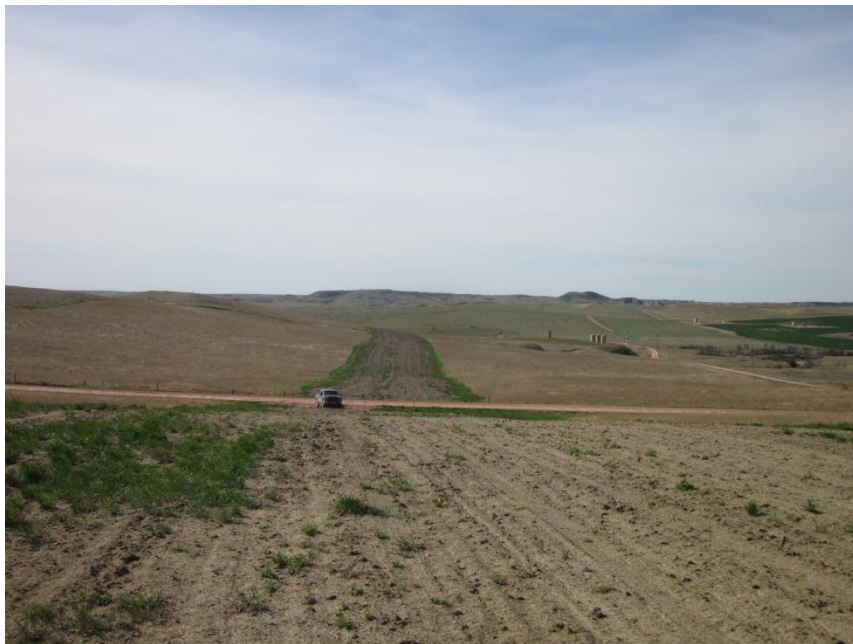
Photo 16. Direction: South. Pipeline right-of-way. Roadway was bored and in good condition.
