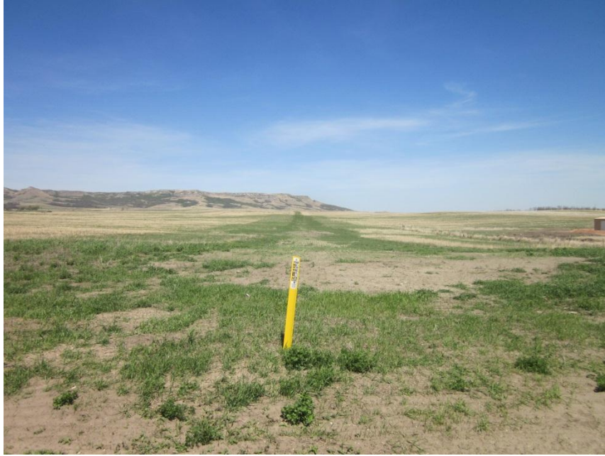
Photo 43. Direction: North. Pipeline right-of-way. Vegetation appeared to have reclaimed some areas.
