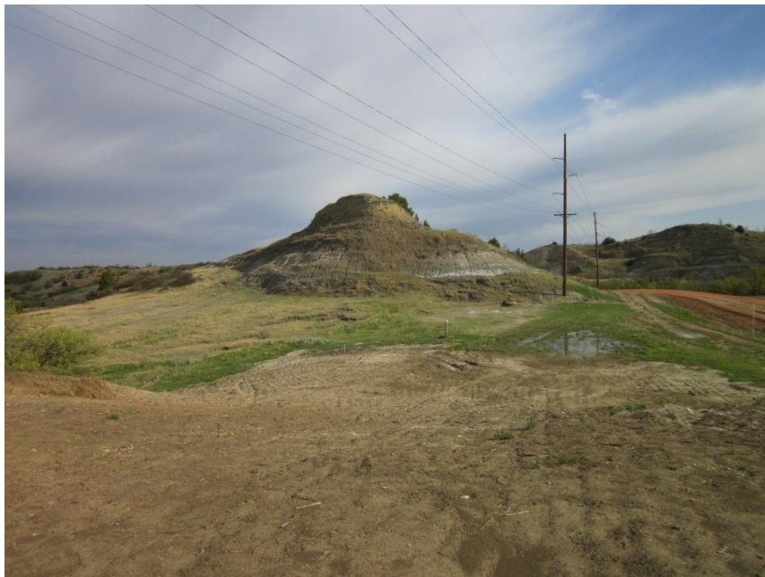
Photo 66. Direction: North. South of where Bridger’s pipeline bores under a badland butte.
