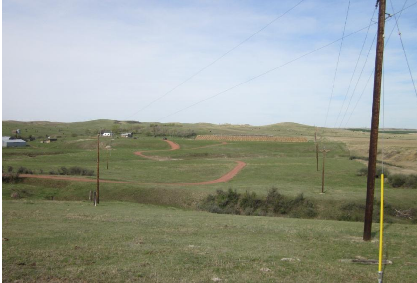
Photo 9. Direction: West. Photo shows a scoria access road constructed for Bridger’s pipeline. The road was well maintained and in good condition.
