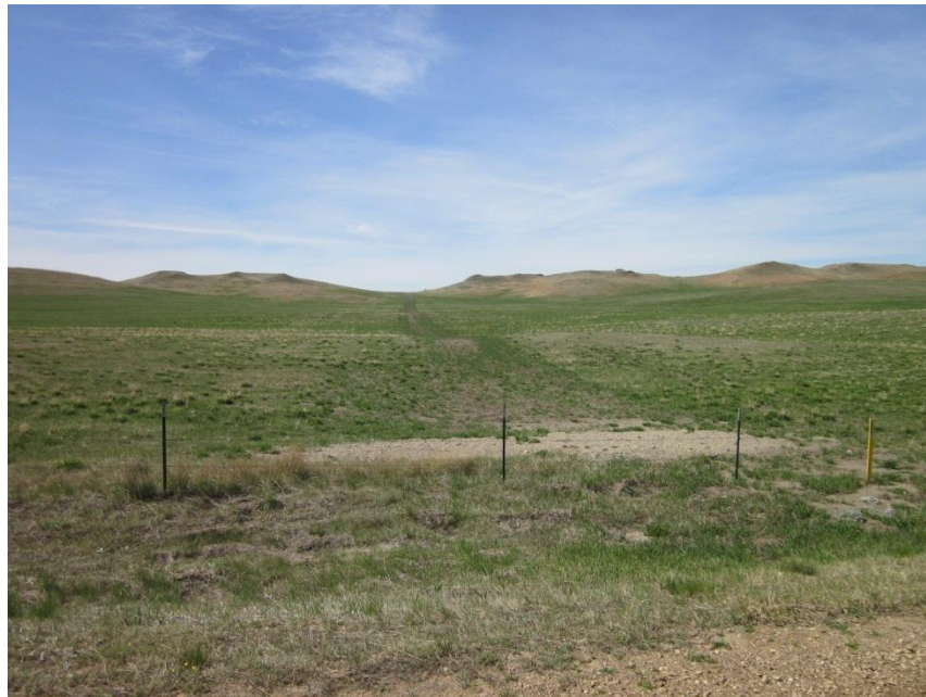
Photo 32. Direction: South. Pipeline right-of-way. This area was nearly completely reclaimed by vegetation.
