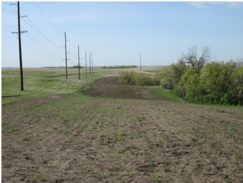
Photo 64. Direction: South. Pipeline right-of-way. Disturbance to the woody area was minimal and the corridor limited to 50ft.
