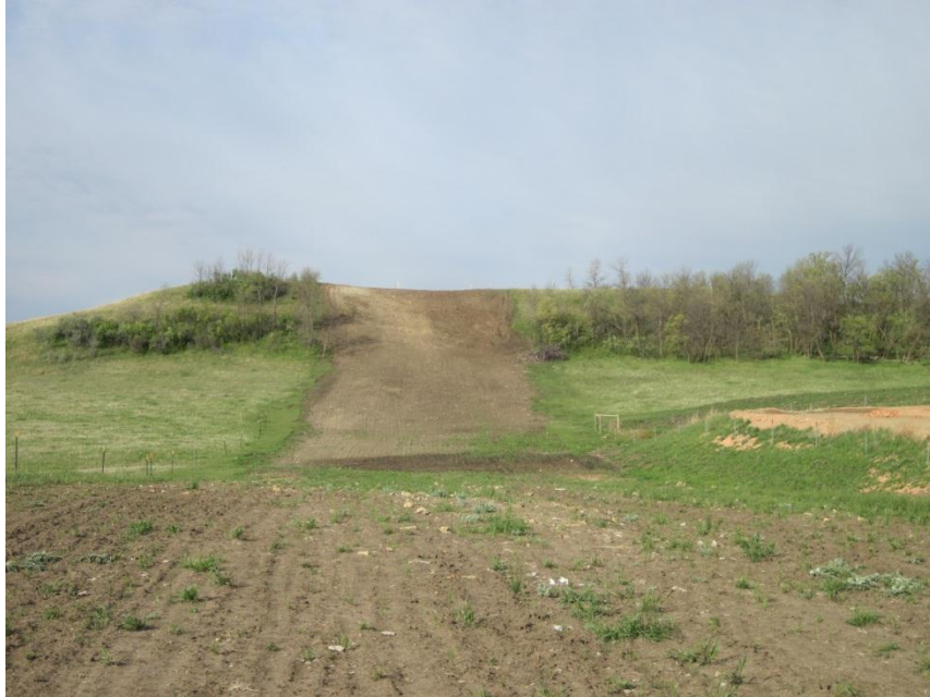
Photo 65. Direction: West. Photo shows the right-of-way of Bridger’s pipeline routing through a wooded area. The cut appeared to have been limited to 50ft.
