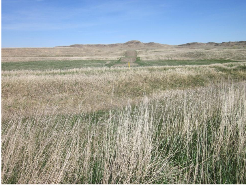
Photo 29. Direction: North. North of where Bridger’s pipeline bored under the Knife River. No erosion or sedimentation to the waterbody was evident.
