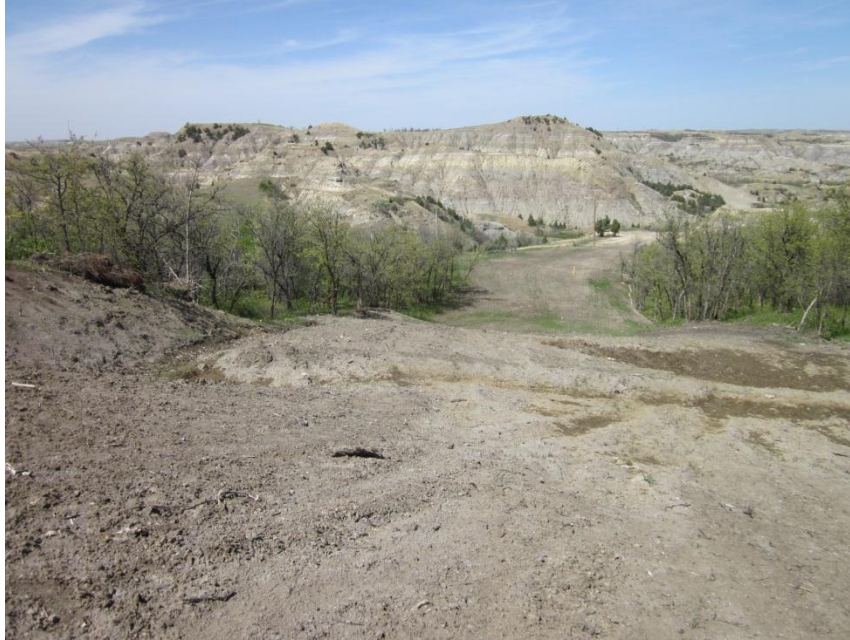
Photo 53. Direction: South. Pipeline right-of-way. Drainage problems caused major erosion in this area last year. Restoration by hauling in soil and channeling water (Photo 54) through the area appeared to have controlled erosion.
