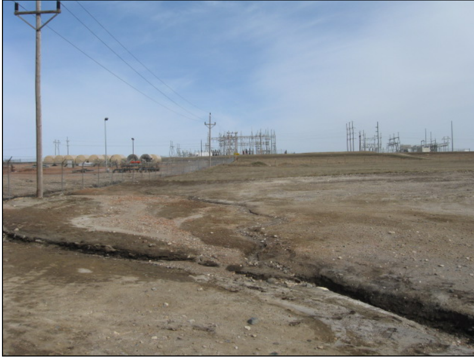
Photograph 5. Hess Footprint property, view facing north.
