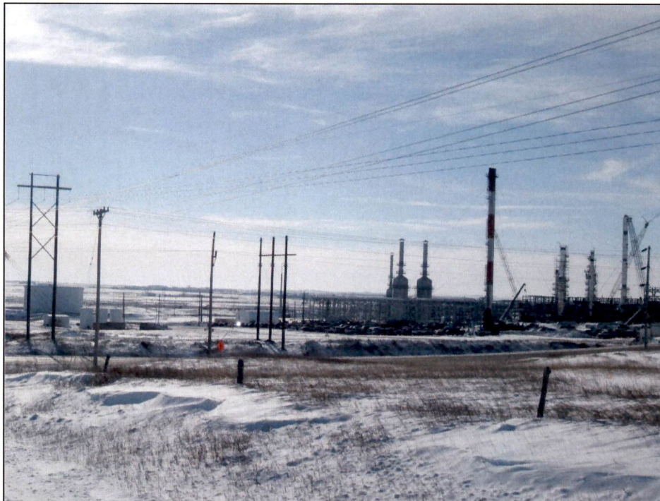
Figure 1. Hess TGP Expansion overview. Photo taken northeast of site facing south-southwest.
