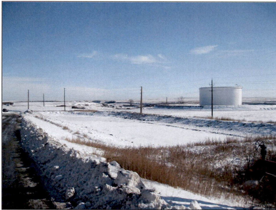
Figure 4. Storm water retention pond #3 located on south side of expansion site. The pond is rock rip-rapped with two inlet culverts from the construction site. The pond is also equipped with an evacuation pump system (pictured in lower right) and an emergency spillway for major runoff event.
