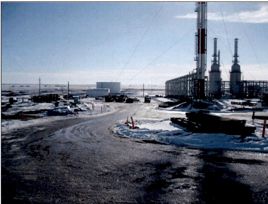
Figure 6. Photo taken facing south near the center of the TGP Expansion.
