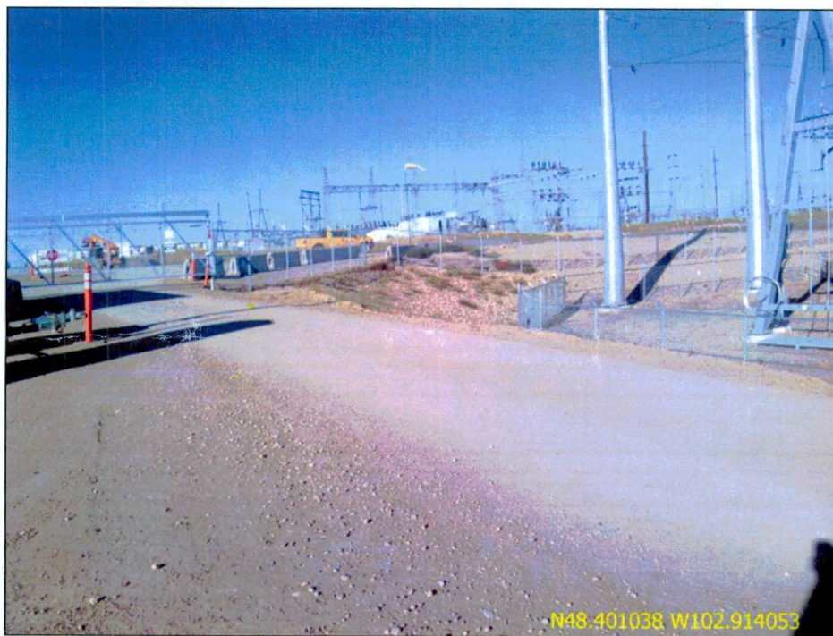
Figure 10. Photo taken facing north at the entrance of the TGP Expansion site. Permanent slopes have been matted and rocked.
