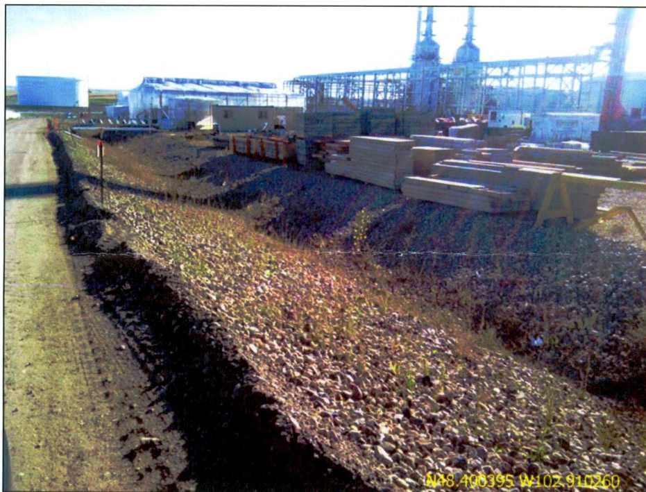
Figure 2. Diversion ditch established at eastern edge of site. Surface water runoff from the site is collected and diverted south to the storm water retention pond through the ditch.
