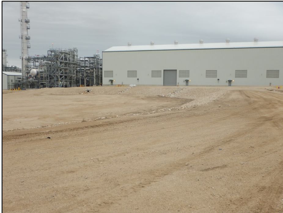
Figure 1. Former temporary workspace east of the TGP Expansion. The perimeter is fenced, equipment removed and level areas have been gravelled.
