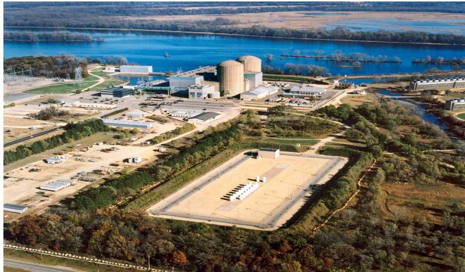
Figure 2: Prairie Island Plant and ISFSI
