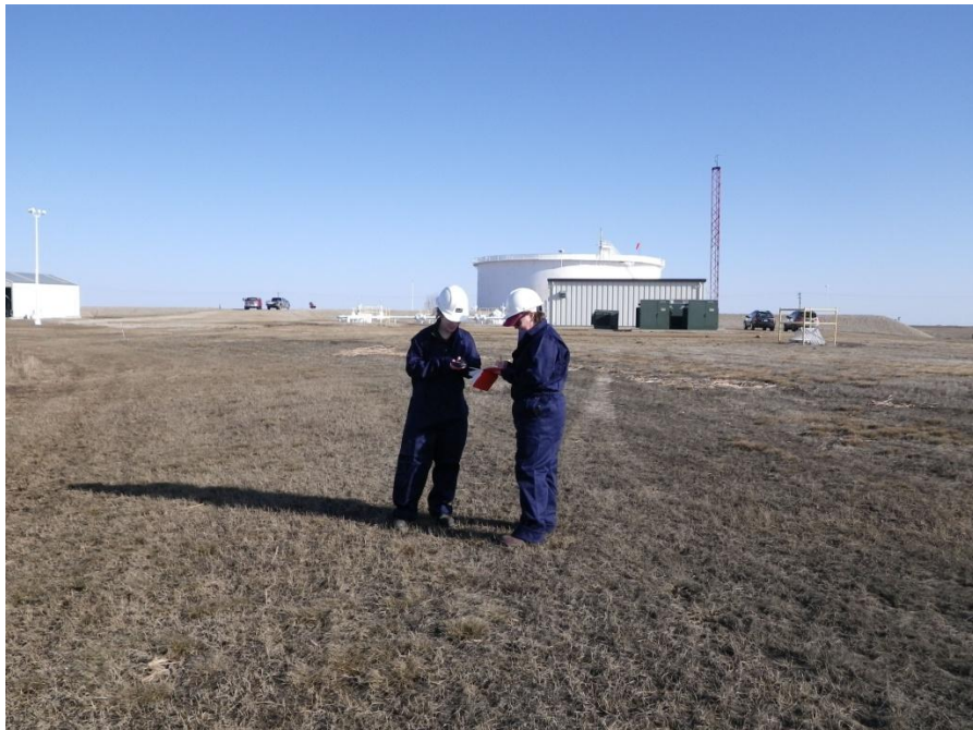
Figure 2: View north over central area in existing Berthold Station (Image #38).
