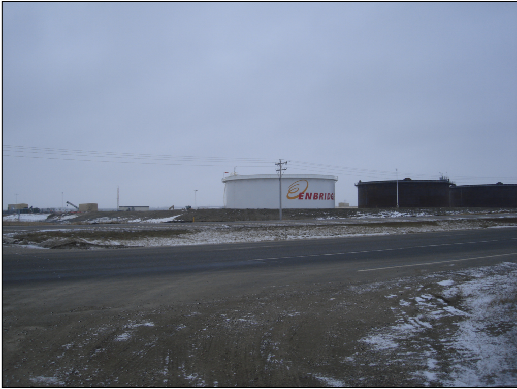
Photo 11. Direction: Southwest. View of the white tank that was rehabilitated as part of this project, the secondary containment berm can be seen around the tank. Additional tanks shown on the right side of the white tank are being added as part of ongoing construction projects.
