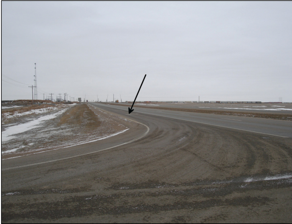
Photo 1. Direction: West. Arrow showing the deceleration and right hand turning lane for eastbound traffic entering the site at the intersection of 296 th St. and Highway 2. Photo also shows road ditches have been graded and reseeded.
