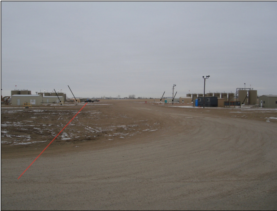
Photo 13. Direction: East. The arrows are showing the location that the 4 inch Enbridge lines terminate and other companies can connect their LACT units, close up can be seen in Photo 16. The red line shows the approximate location of the 10 inch line that the 4 inch lines feed into.
