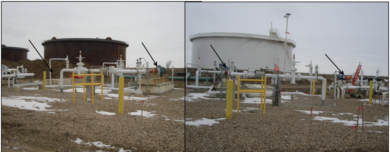
Photo 8. Direction: North/Northwest. Arrow on the far right shows the 50 Hp booster pump. The three arrows on the left show the locations where three positive displacement (PD) pumps had been installed, two of those PD pumps were part of this project and the third PD pump was part of the PU-10-564 project. The two PD pumps for this project were replaced by the centrifugal pump shown by the second arrow from the right.
