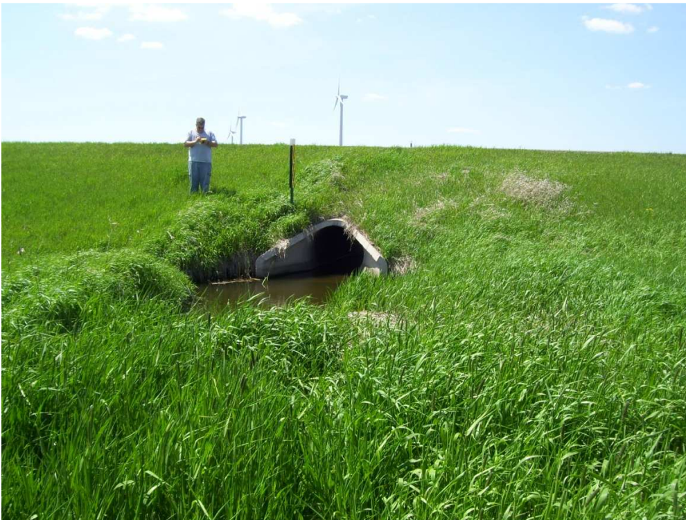
Location 142-57-15-2: View West 05-18-10
