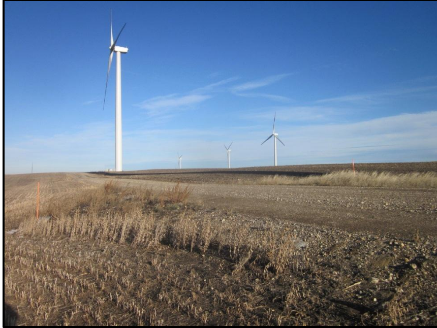
Photo 19. Direction: Southeast. Access road between Turbines 253 and 252, showing culvert in place (red markers) and adjacent cropland.
