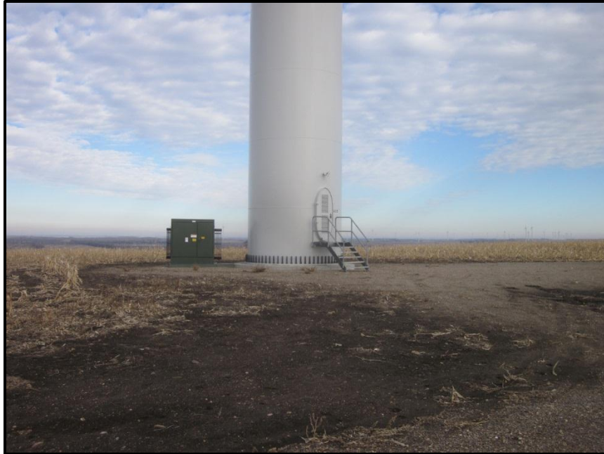
Photo 5. Direction: North/Northeast. Close-up of base of Turbine 273, showing pad-mounted transformer to the left and gravel pad surrounding tower. The crop remnants did not indicate any problematic areas or reclamation issues.
