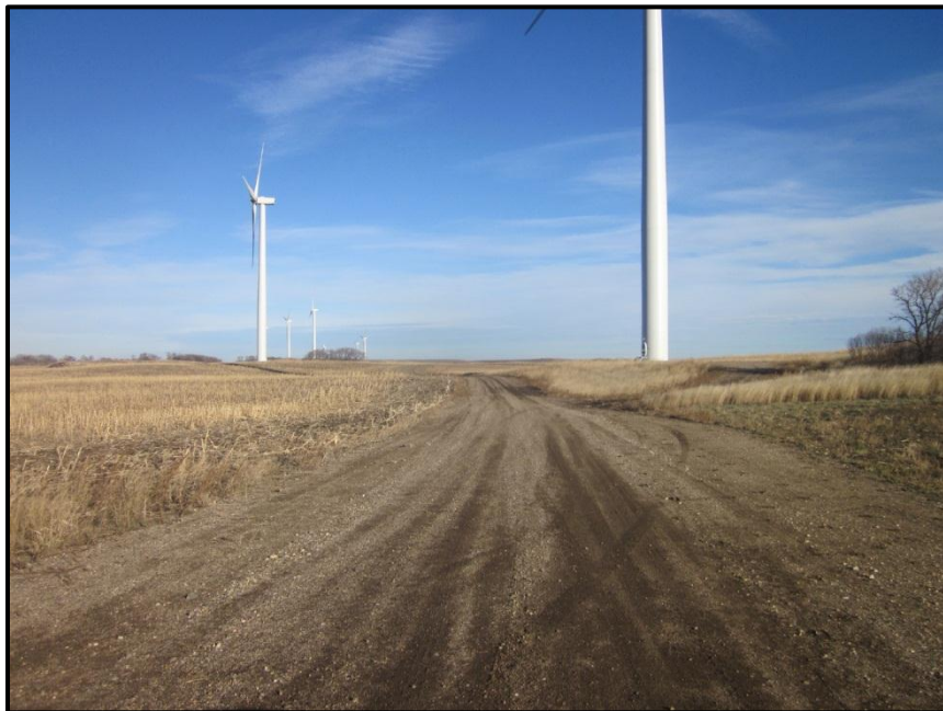
Photo 16. Direction: Northeast. Access road entrance to Turbines 246-247. Proper signs were in place. Cropland, roads, and towers were in good condition. The road near Turbine 247 in the distance had been adjusted to avoid a wetland basin.
