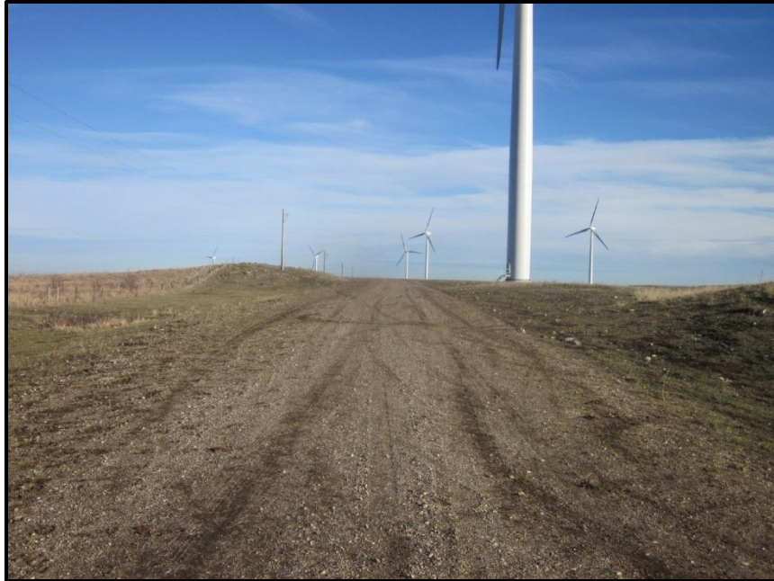
Photo 17. Direction: East. Access road entrance to Turbines 248-250. The edges of the road had been reclaimed but the dense growth of seeded grasses typical of other areas was not present here. This could have been due to the heavy grazing in this pasture.
