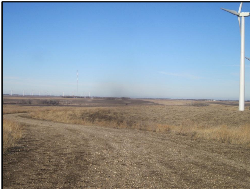
Photo 18. Direction: North. Access road near Turbine 249 (on right). The road and adjacent collection line was routed to the west around an archeological site (32BA197) on the hilltop shown in the center.
