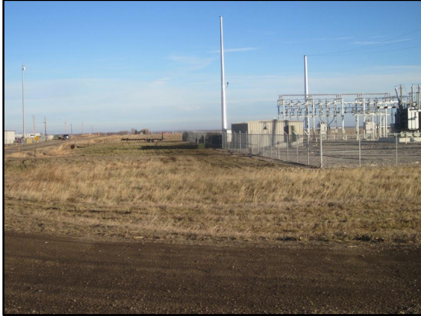
Photo 3. Direction: East. View of the area to the north of the new substation, showing the established vegetation.
