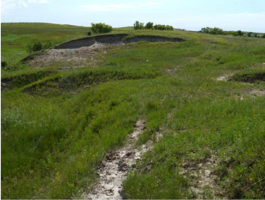
Figure 16 Cutbank in the northeast portion of 32MZ303, view to the southeast (image 7-23-11-8896).
