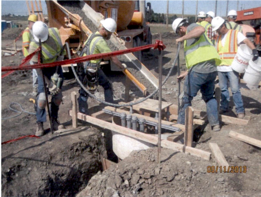
115kV piers concrete placement (looking NW)
