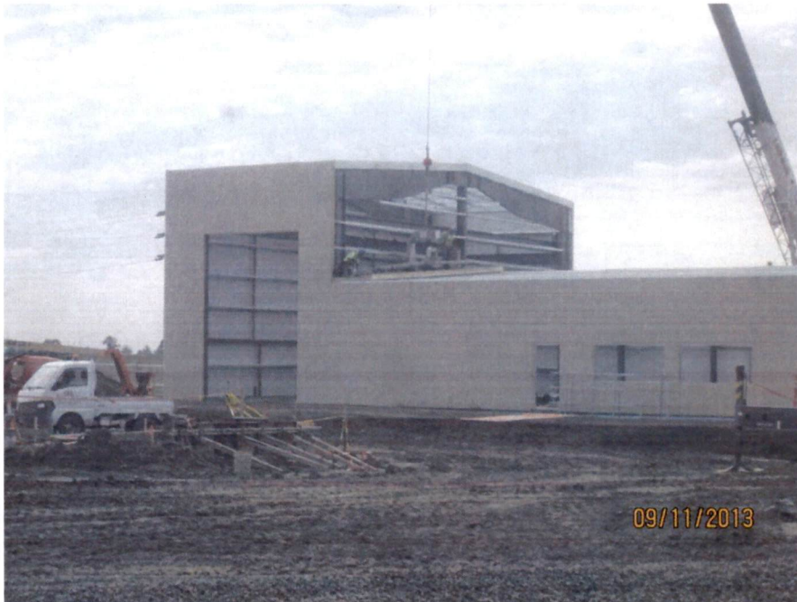
Service Building roof sheeting installation (looking SE)
