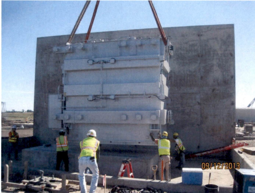
GSU transformer installation (looking S)
