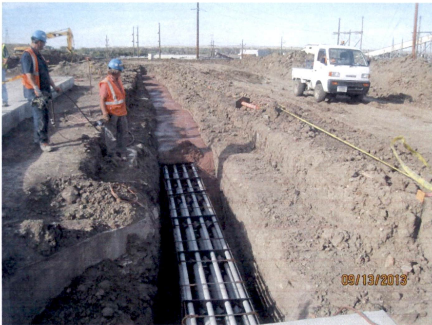
Duct bank concrete installation (looking N)
