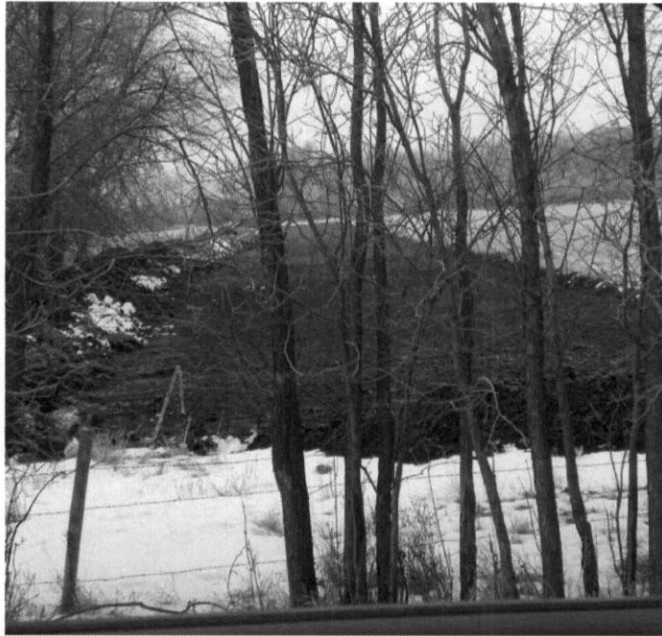
Photo 4: Looking west from 157 th Ave NW/34 th /156 th ; ROW clearing has occurred, no construction, ROW staking present.
