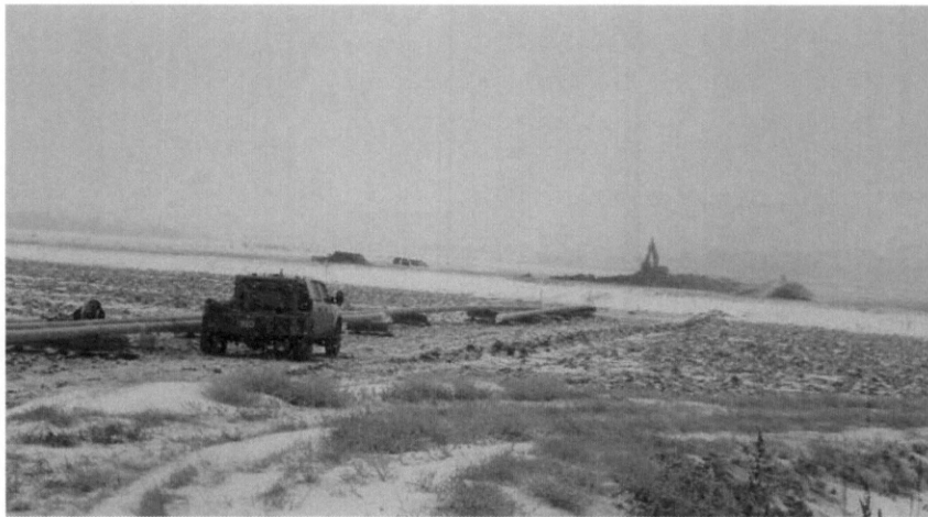
Photo 1: Looking southwest from 36 th ST NW at Project ROW, notice pipe strung in preparation installation via open trench method.
