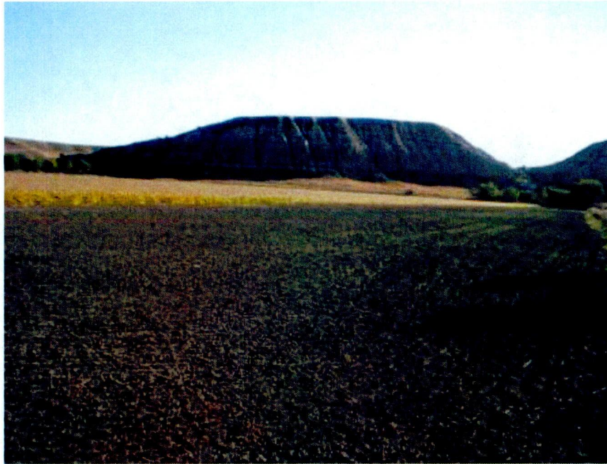
Image 4: Entry point for Yellowstone River HDD, area has been returned to agricultural use.
