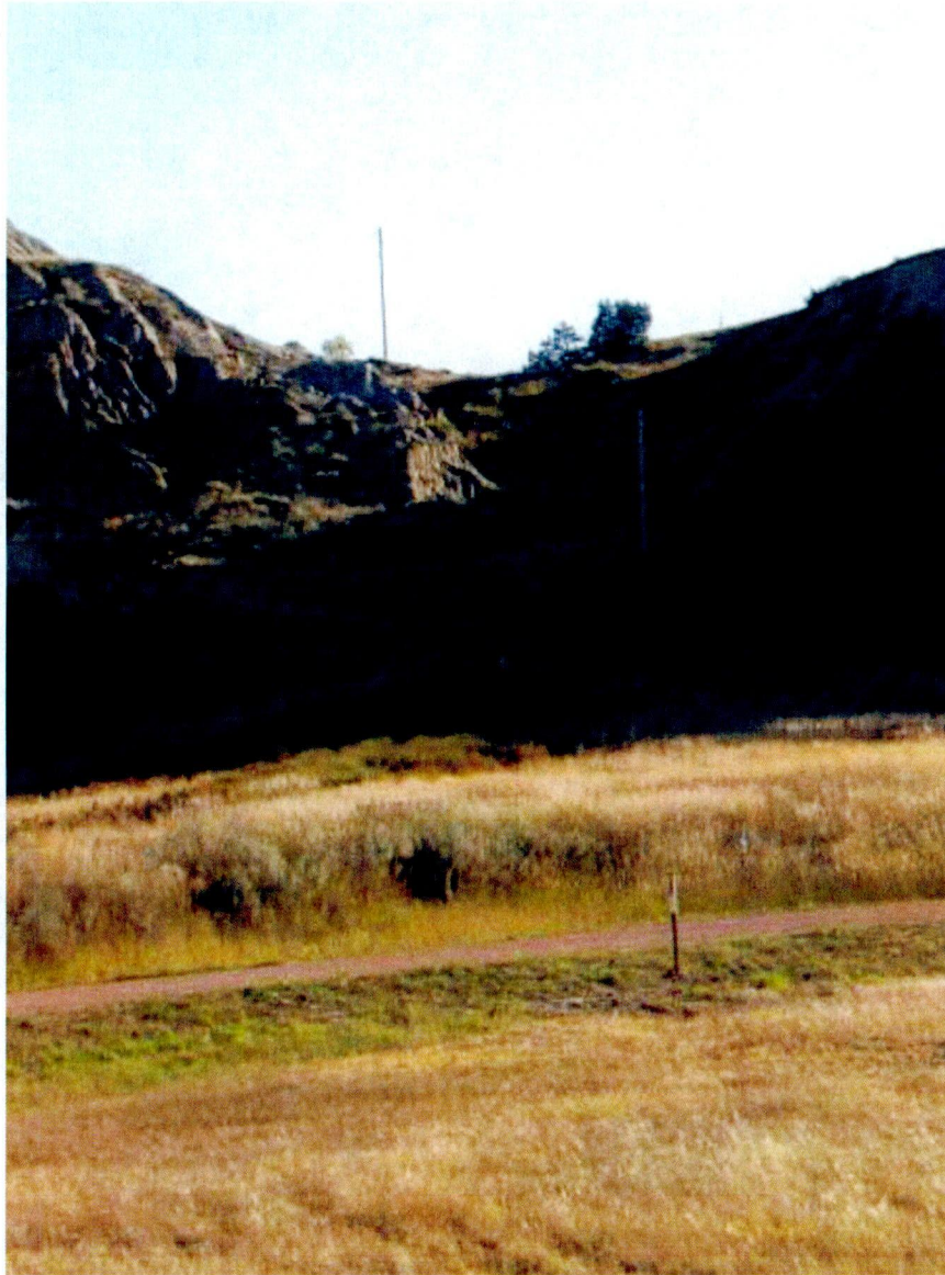
Image 3: Looking east at hillside HDD to avoid impacts to protected plant. No issues or concerns, preconstruction contours and conditions preserved.
