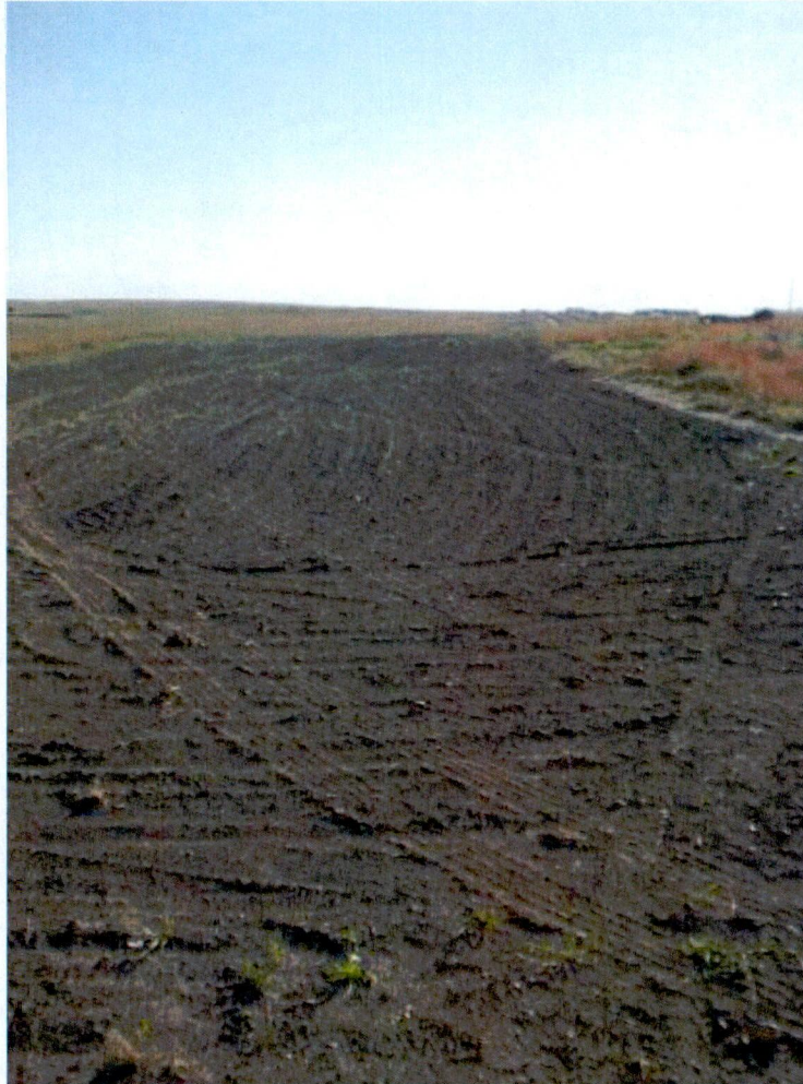
Image 6: ROW near Hiland Plant, ROW has been returned to pre-construction contours and land use, re-vegetation is underway, continue to monitor until 70% ground cover is achieved.
