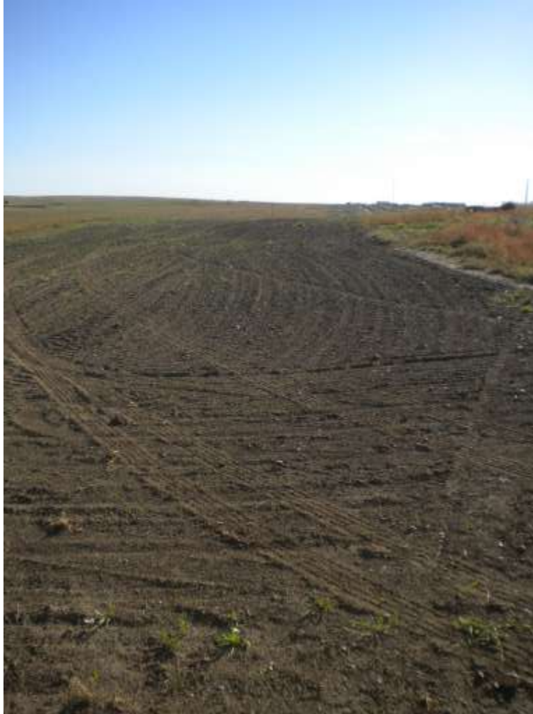
Image 6: ROW near Hiland Plant, ROW has been returned to pre-construction contours and land use, re-vegetation is underway, continue to monitor until 70% ground cover is achieved.
