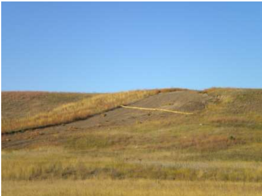
Image 5: Looking back at ROW in Section 31, erosion control measures properly placed and in good working order, regrowth of vegetation is underway. Continue to maintain erosion control measures until re-vegetation reaches 70%.
