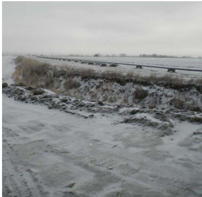
Photo 3: Looking east at pipe strung for HDD of irrigation channels and existing creek and ditches.
