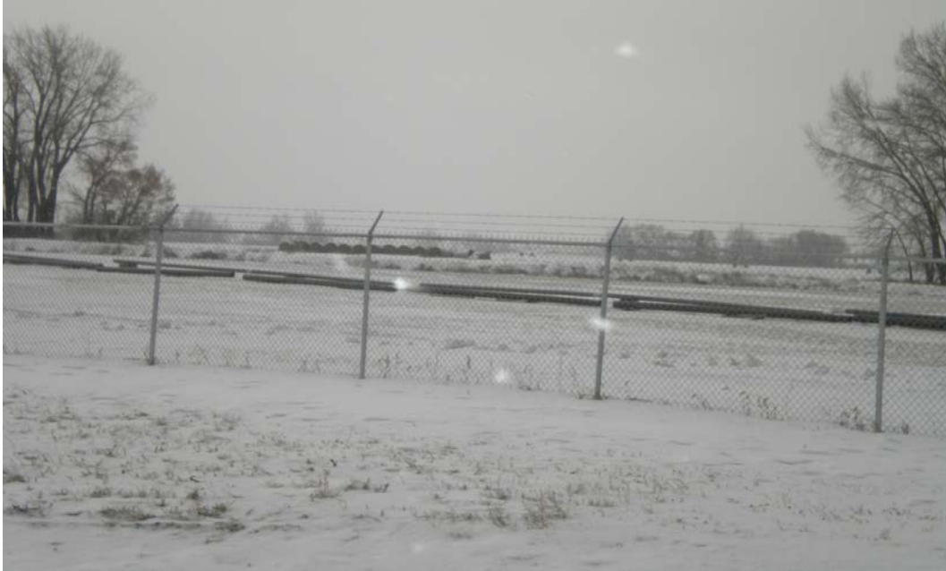
Photo 2: Looking south from Hiland Rail Terminal at pipe strung for Hwy 58 and BNSF Railroad HDD and installation of pipeline into facility.
