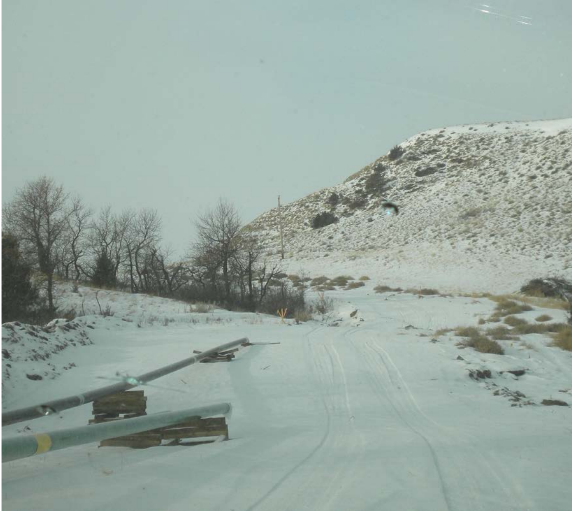
Photo 5: Looking west from Project ROW just north of 36 th Street NW; orange 3 piece flags mark entrance/exit points of planned HDDs to avoid trees, cultural site and protected plant. The majority of this hill will be HDD to avoid the rough terrain including the aforementioned sensitive features. No Trees will be removed during construction.
