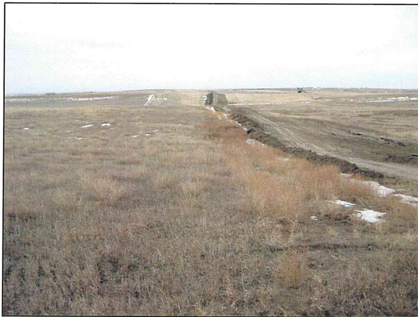
Photo 2. Taken facing west from the section line between Sections 6 and 1. The ROW has been reseeded (decadent alfalfa and smooth brome) and can be seen just south of the topsoil windrow.
