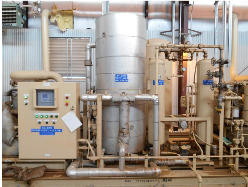
Picture 11 Instrument Control Air
