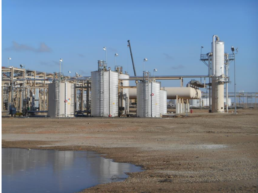
Picture 3 Storage Tanks
