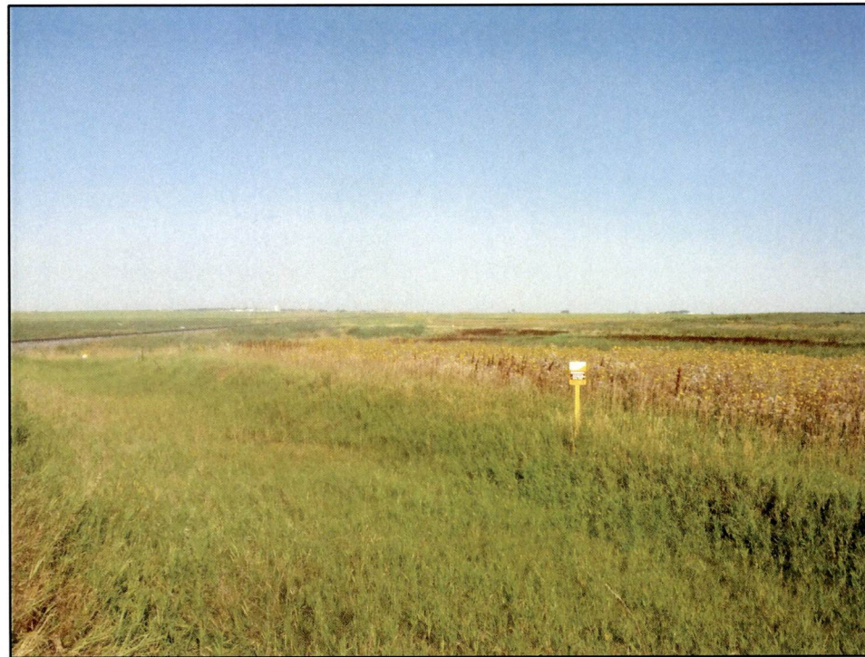
Photo 10. Station 288+00 Looking northwest at a horizontally directionally drilled wetland.
