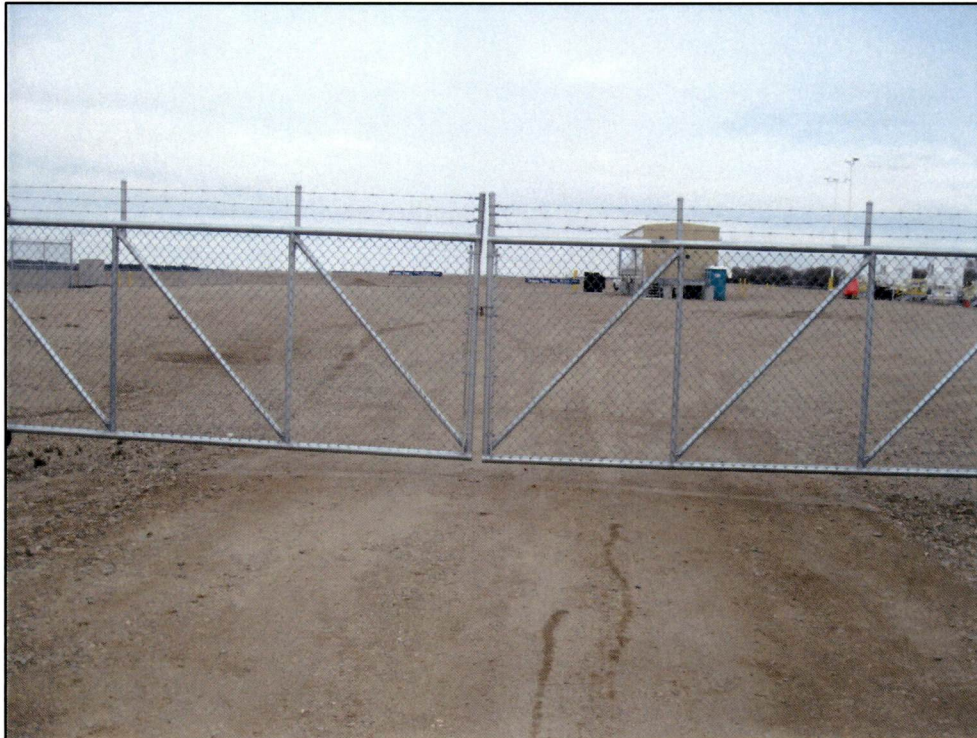
Photo 18. Gates at Kenaston Pump Station
