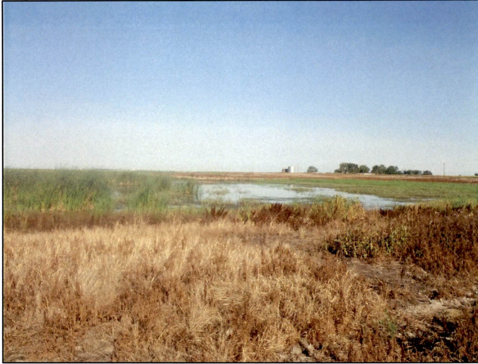
Photo 11. Station 308+00 Looking northwest at a directionally drilled wetland.
