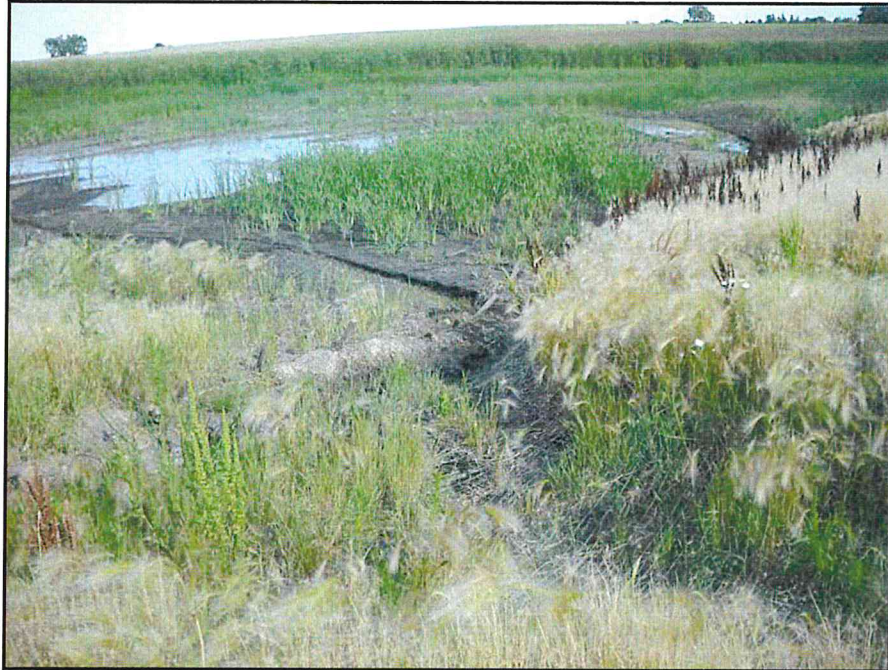
Photograph 5. An erosion area located near the retention pond at the end of the storm water drain has cut through the upland buffer and washed sediment into the mitigation wetland.
