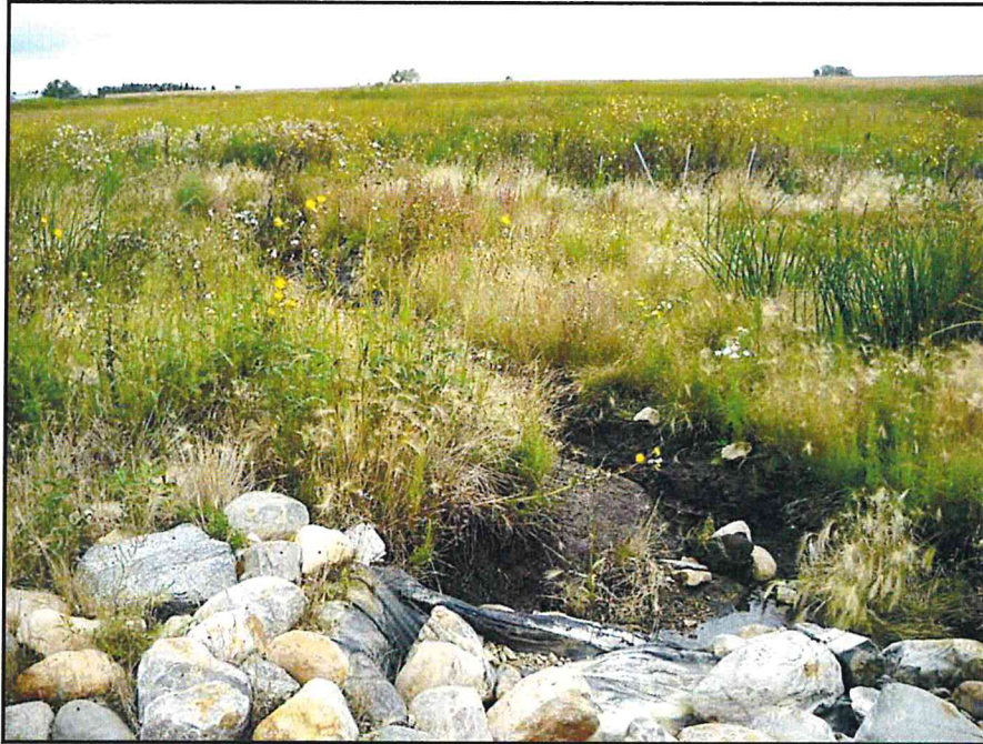
Photograph 8. An erosion area located near the retention pond at the end of the storm water drain has cut through the upland buffer and washed sediment into the mitigation wetland.
