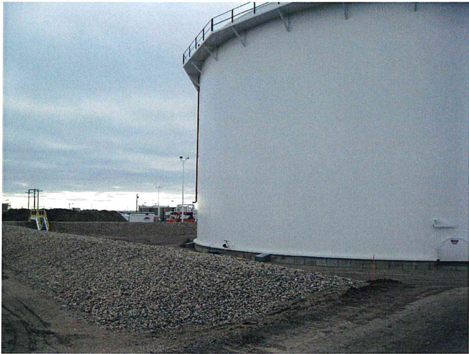
Figure 15: New Tank at Berthold Pump Station
