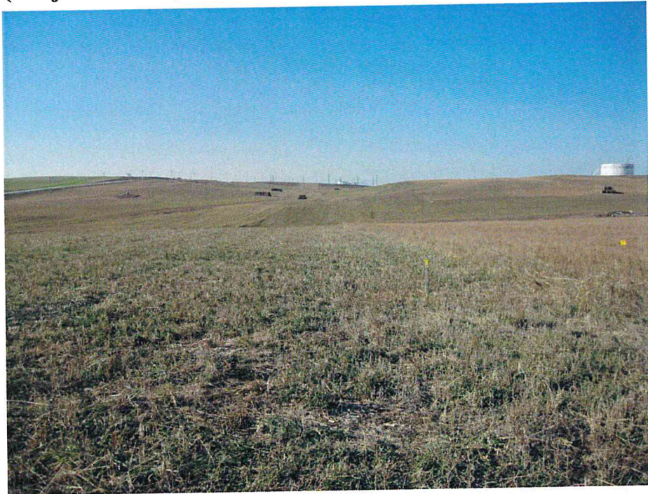
Figure 1: STA 33+00 Looking West at Pipeline Trench (between M.P. 76.1 – 75.3)
