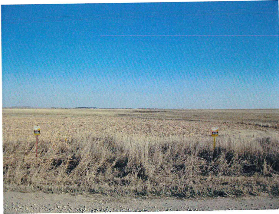
Figure 3: STA 1086+80 Looking East at Pipeline Trench (between M.P. 56.6 – 55.7)
