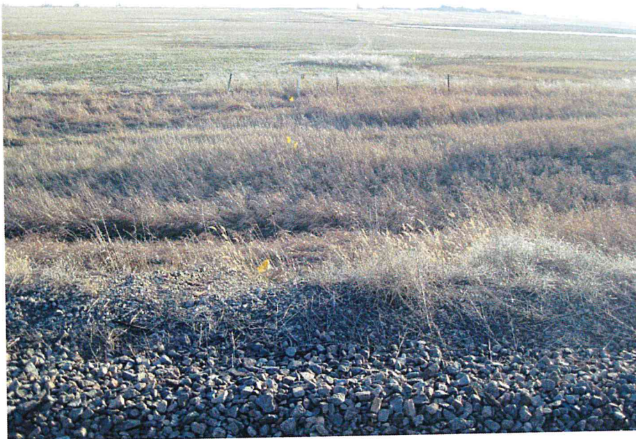
Figure 10: STA 1406+00 Looking South at Pipeline Trench (between M.P. 26.6 - 25.8)
