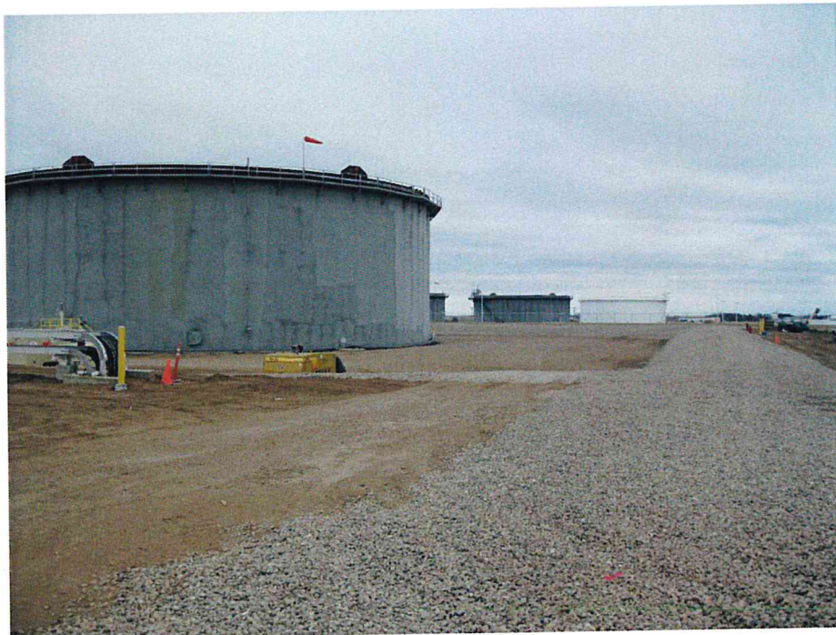
Figure 14: New Tank at Berthold Pump Station
