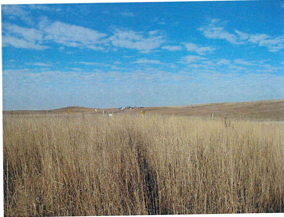
Figure 5: STA 202+00 Looking West at Pipeline Trench (between M.P. 47.6 – 47.1)
