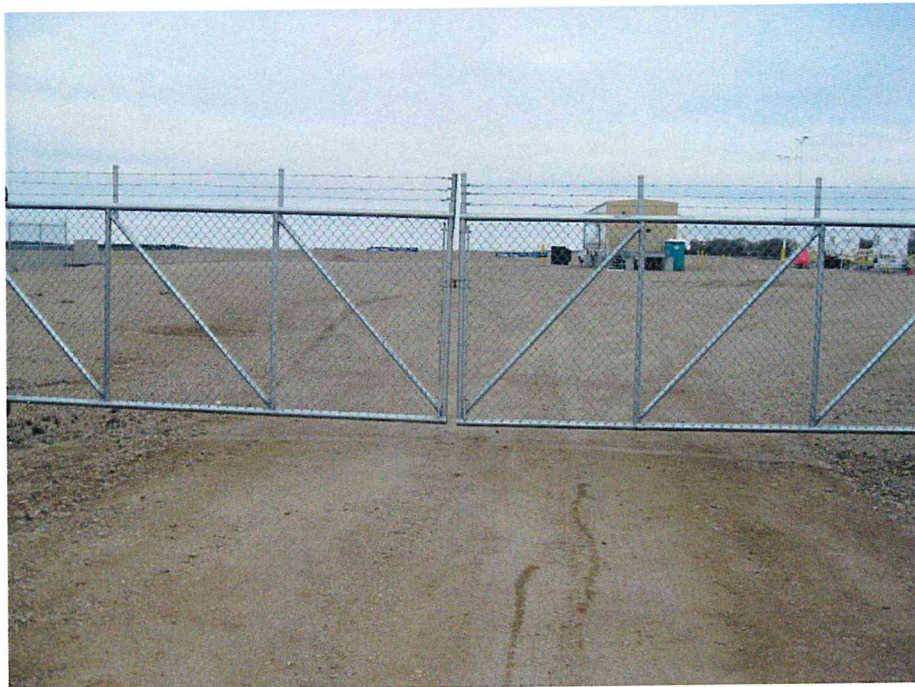
Figure 26: Gates at Kenaston Pump Station
