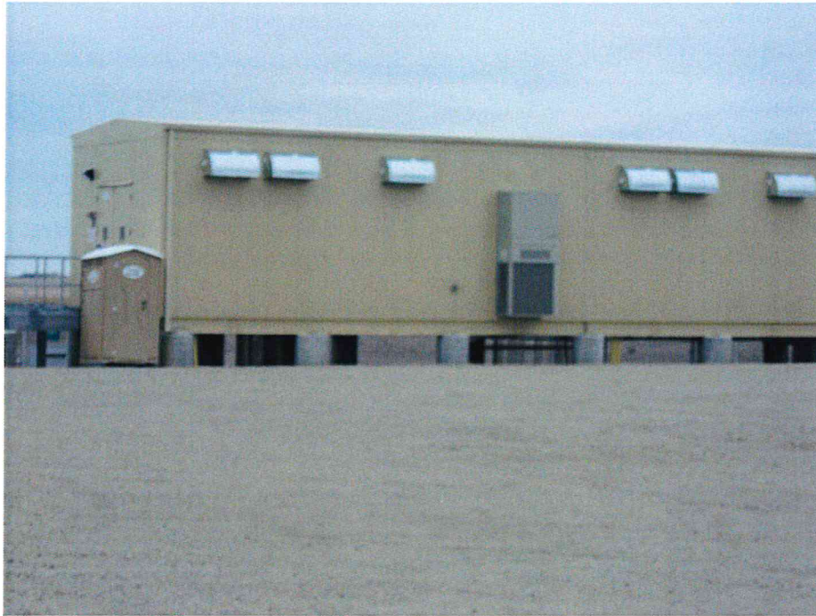
Figure 21: Electrical Equipment Building at Beaver Lodge Pump Station
