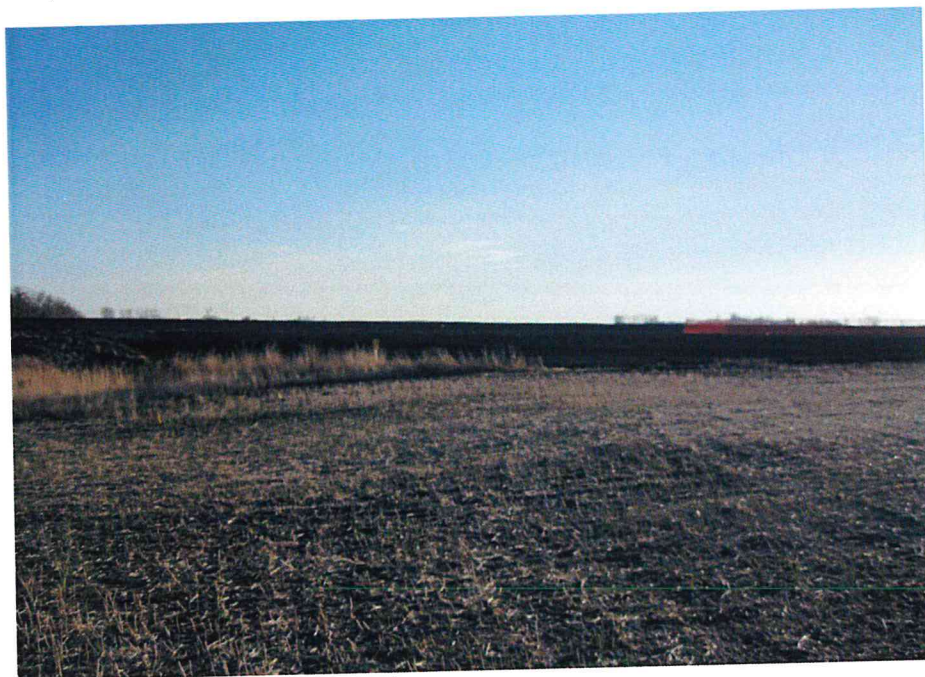
Figure 8: STA Looking East at Pipeline Trench (between M.P. 30.2 - 29.3)
