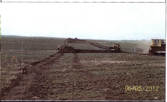
Stripping TopSoil
