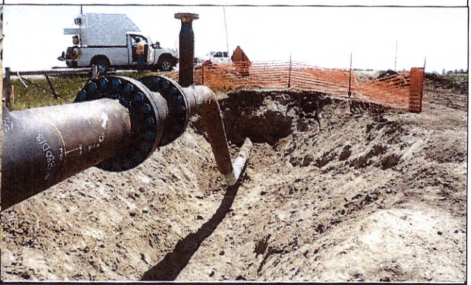
Tie In / Williams Co ND
