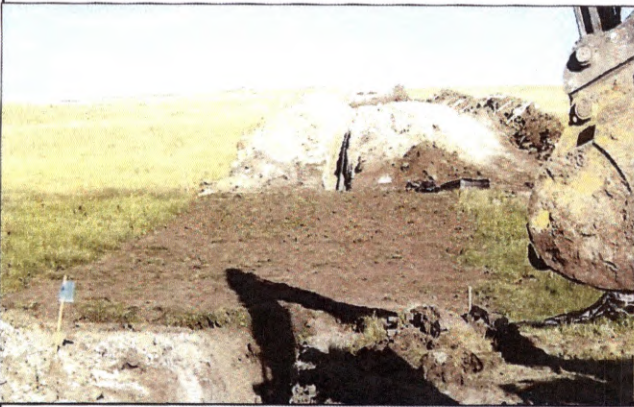
Tie In / Williams Co ND
