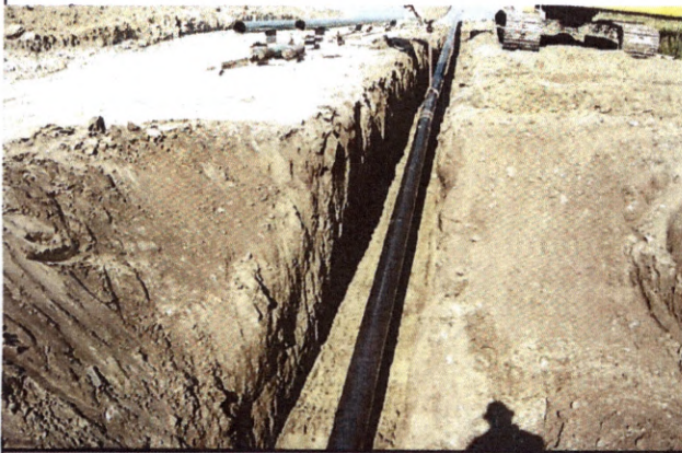
Pipe lowered in ditch.
