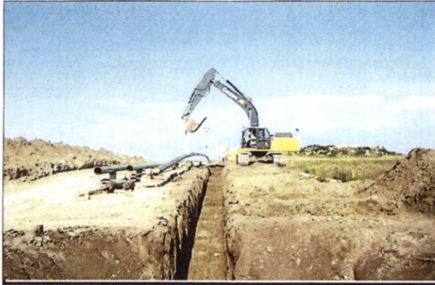
Ditch Line ready for lowering in.
