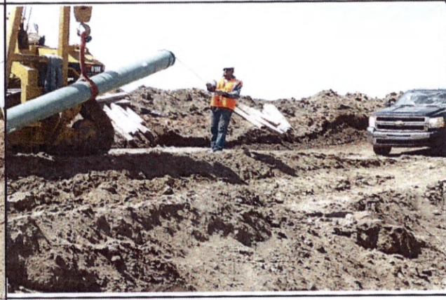
Lowering pipe in ditch
