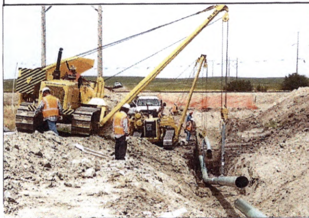
Lowering pipe in ditch
