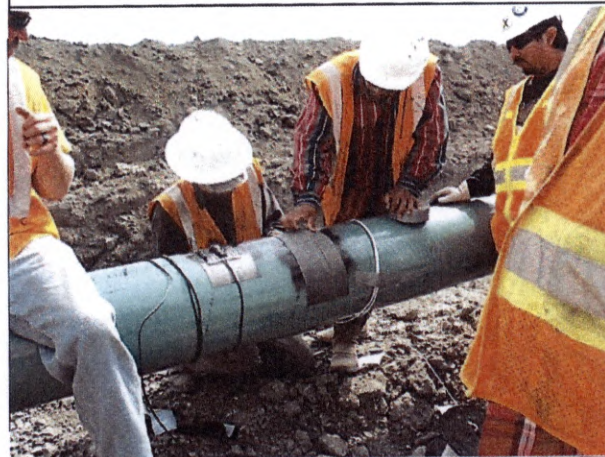
Installing Test Leads
