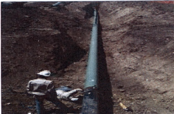
Welding line pipe to bore pipe.
