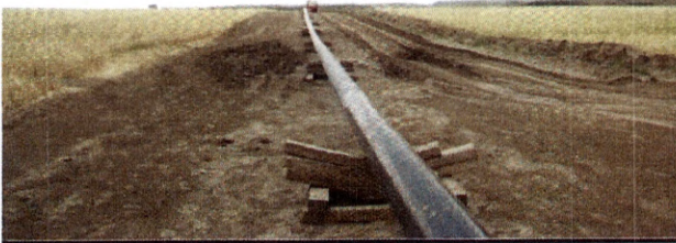
Pipeline laid and welded
