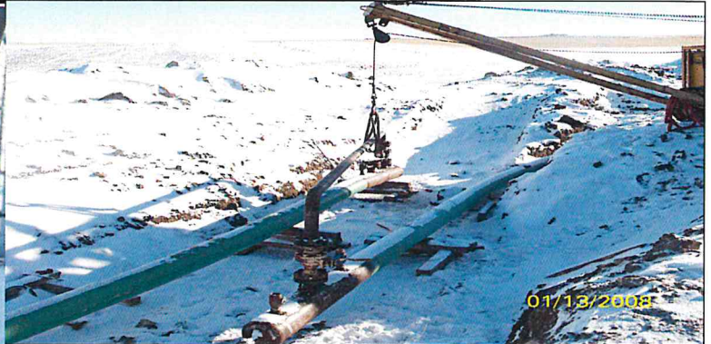
Jumper at G3 for Hydro test
