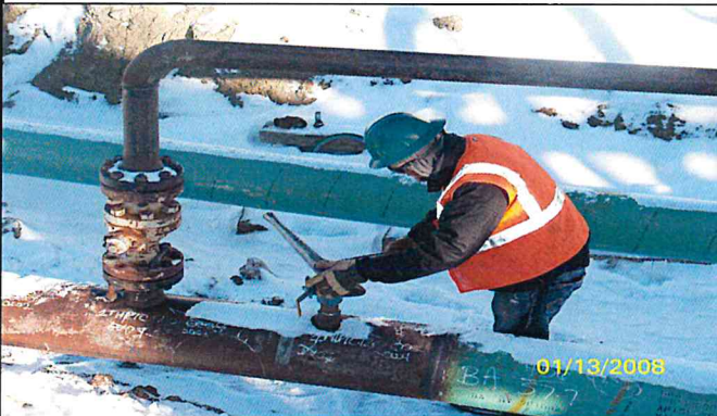
Jumper @ G3 and relief valve installation
