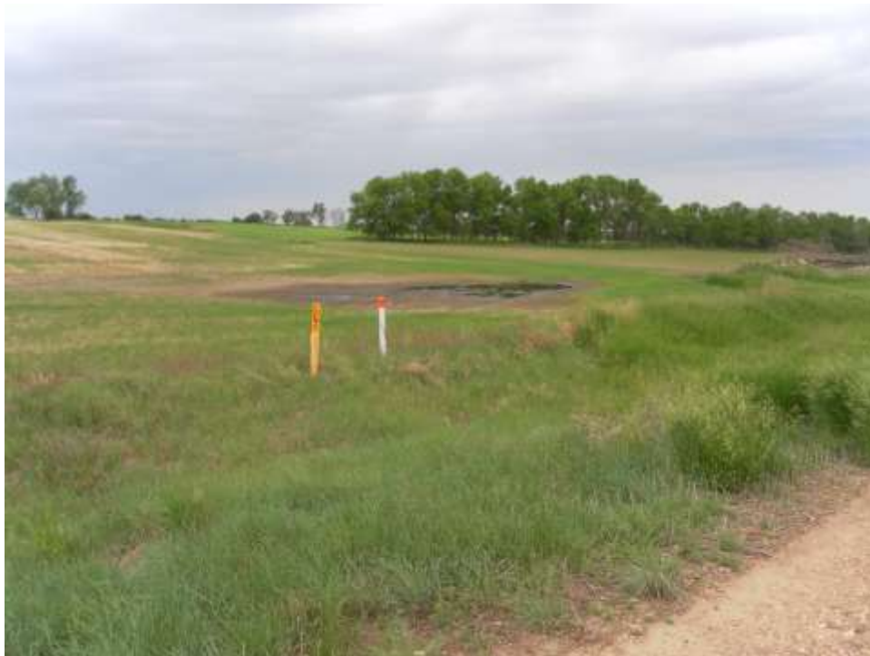
Photo 4 – Typical pipeline markers at road crossing
