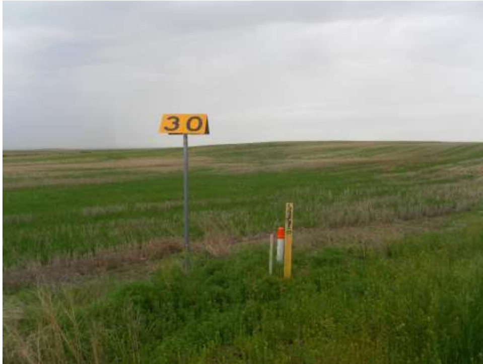
Photo 5 – Typical pipeline markers at road crossing
