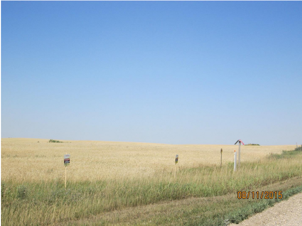
Photo 9 – Typical pipeline markers showing Enbridge’s paralleling line.
