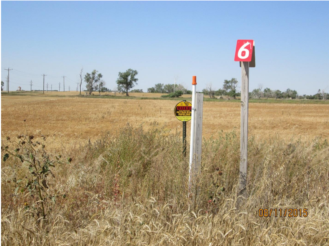
Photo 6 – Typical pipeline marker. Note pipeline markers going through tree row in background.
