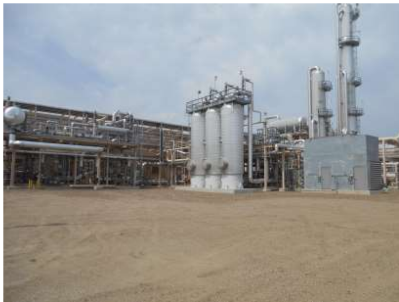
Picture 2 Fractionator Column
