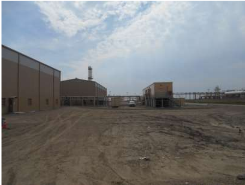
Picture 7 Compressor Buildings
