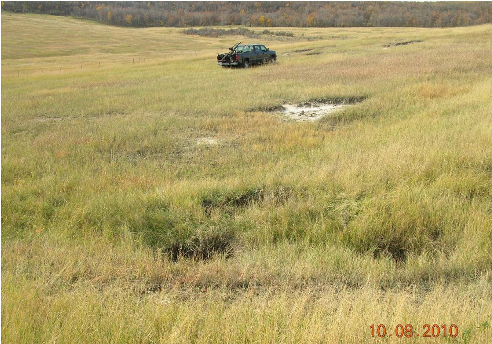
Figure 6. Erosion and piping near the permit boundary in the SE 1 / 4 of the SE 1 / 4 of the SW 1 / 4 and the SW 1 / 4 of the SW 1 / 4 of the SE 1 / 4 of Section 31 (Tract 4C) south-southeast of soil probe number 51.
