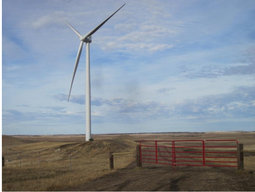
Photo 5. Direction: Northwest. View from the access road to Structure 215. Note repaired fence and new access gate.
