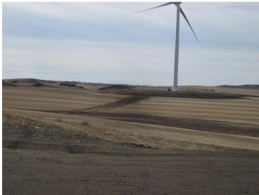
Photo 6. Direction: Southwest. From the pad of Structure 209, view shows feeder line scars leading to Structure 210. Reclamation of this area was still ongoing. Other areas where feeder line scars had been reclaimed appeared in good condition, with no impacts to agricultural production.
