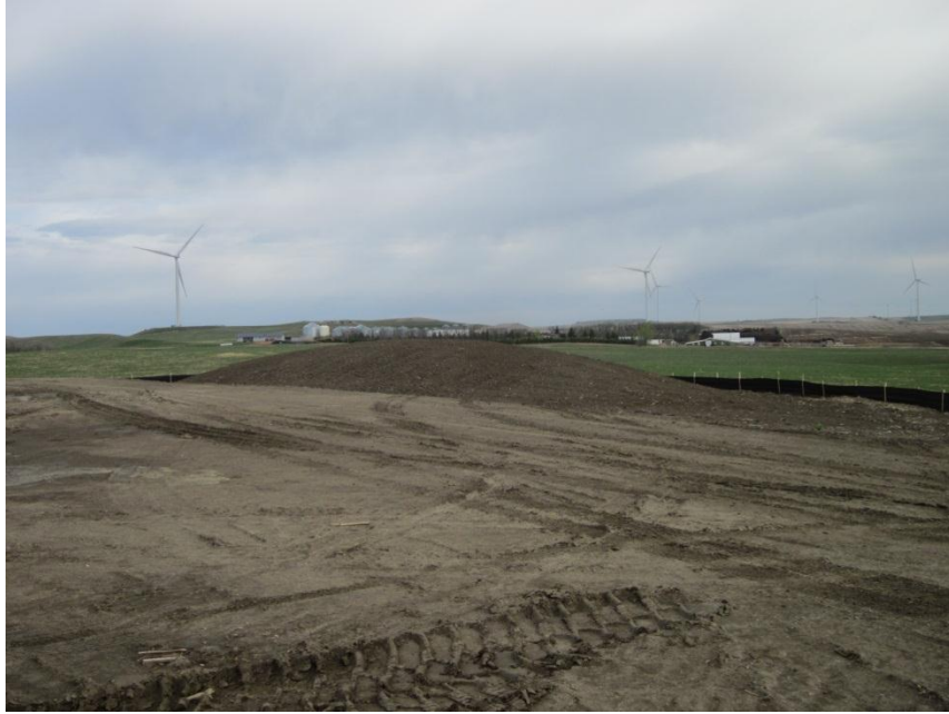
Photo 11. Direction: South. Example segregated topsoil pile at Structure 212 observed during the interim inspection. All topsoil was mounded on site, with appropriate erosion controls at all structure locations.
