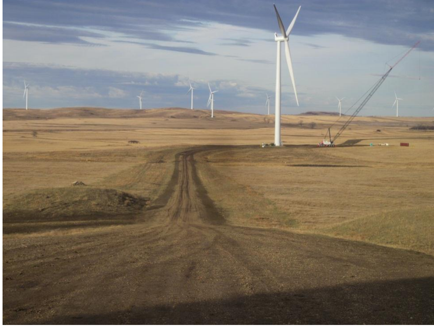
Photo 1. Direction: West. View from the access road to Structure 206 (shown, south of crane) and 207 (not shown). Topsoil had been segregated and replaced as evidenced by successful establishment of vegetation. Revegetation along roads was well established, and native species appeared to have been used.
