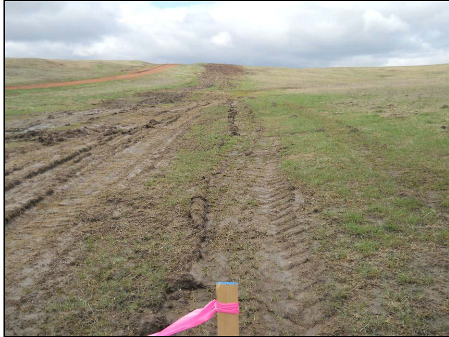
Figure 2. Existing pipeline scar, near milepost (MP) 37.5, facing west.
