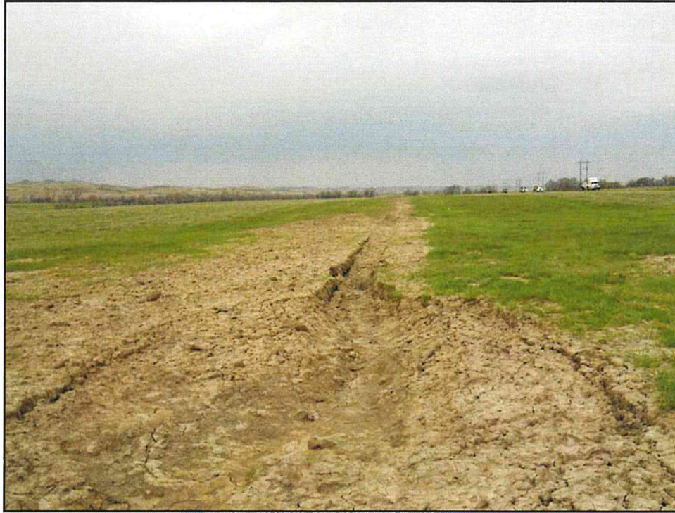
Figure A.1. View of the project co-location alignment. Note existing pipeline disturbance area and agricultural field within the pipeline co-location area.
