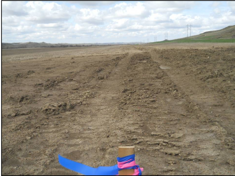
Figure 3. General topography and adjacent agricultural disturbance along the western portion of pipeline corridor, facing west.
