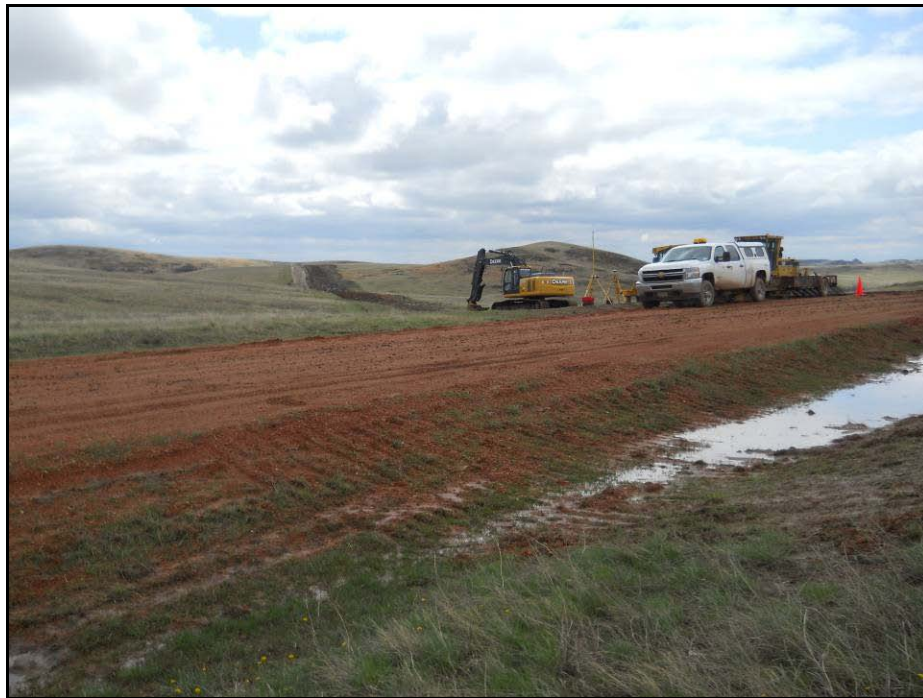
Figure 16. 32MZ168 site overview, showing crowned-and-ditched scoria access road, facing southwest.
