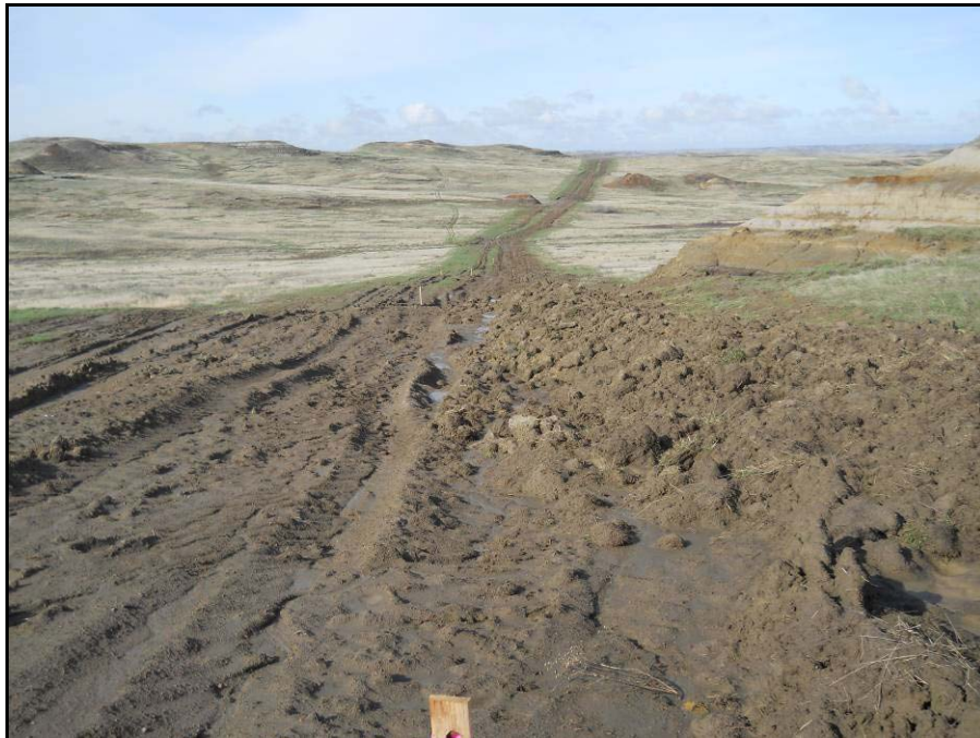
Figure 3. Existing pipeline scar, near MP 40, facing southwest.
