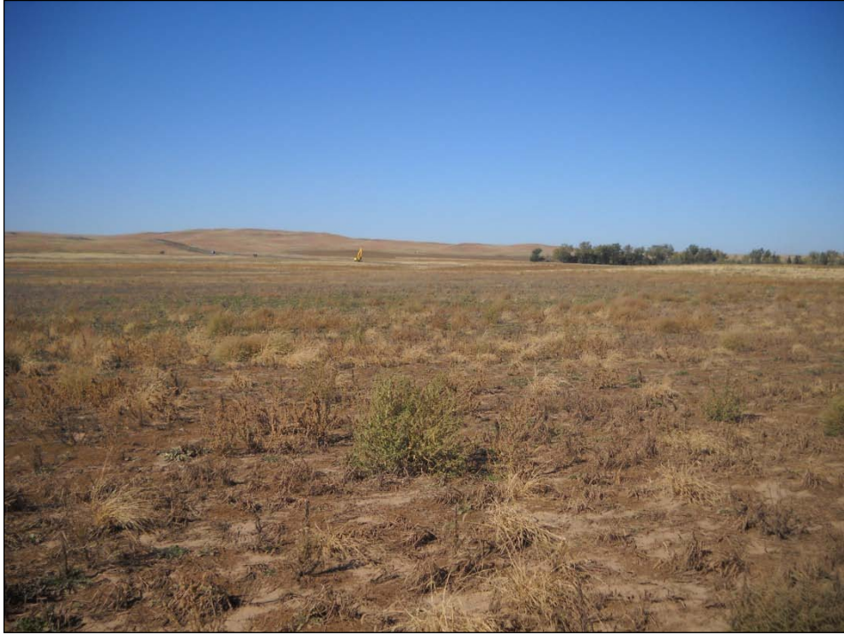
Figure 6. View of northern reroute area from southeastern edge of survey block, construction equipment located within existing pipeline corridor in background, facing northwest.
