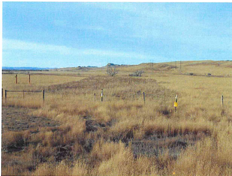
Photo 26 – Direction: Northwest – Showing revegetation near pipeline marker 44. ND 16 Highway crossing.
