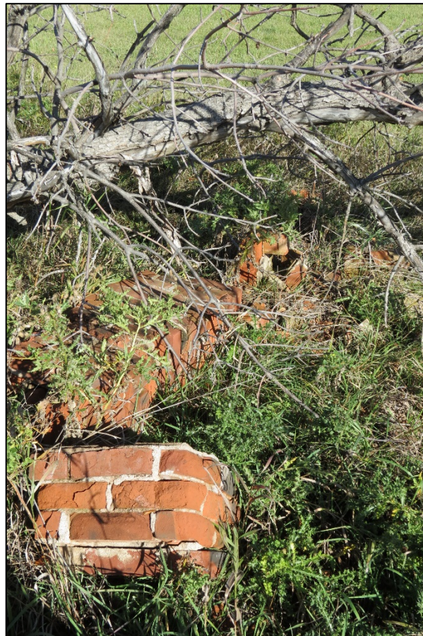
Figure 6-1. Chimney remnants at 32MHXXX, View looking north.
