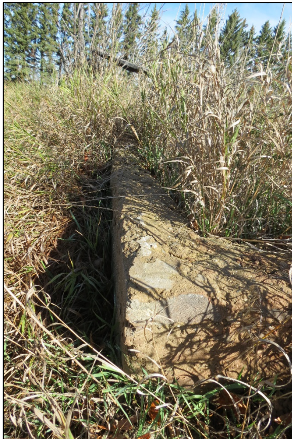
Figure 6-3. Historic foundation at 32MHXXX, View looking north.
