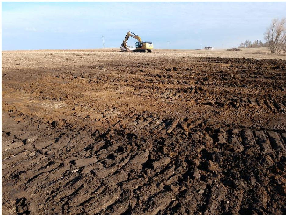
Figure 4. There is a distinct color change between topsoil and subsoil. Subsoil is easily distinguished by dark brown, clay soils.
