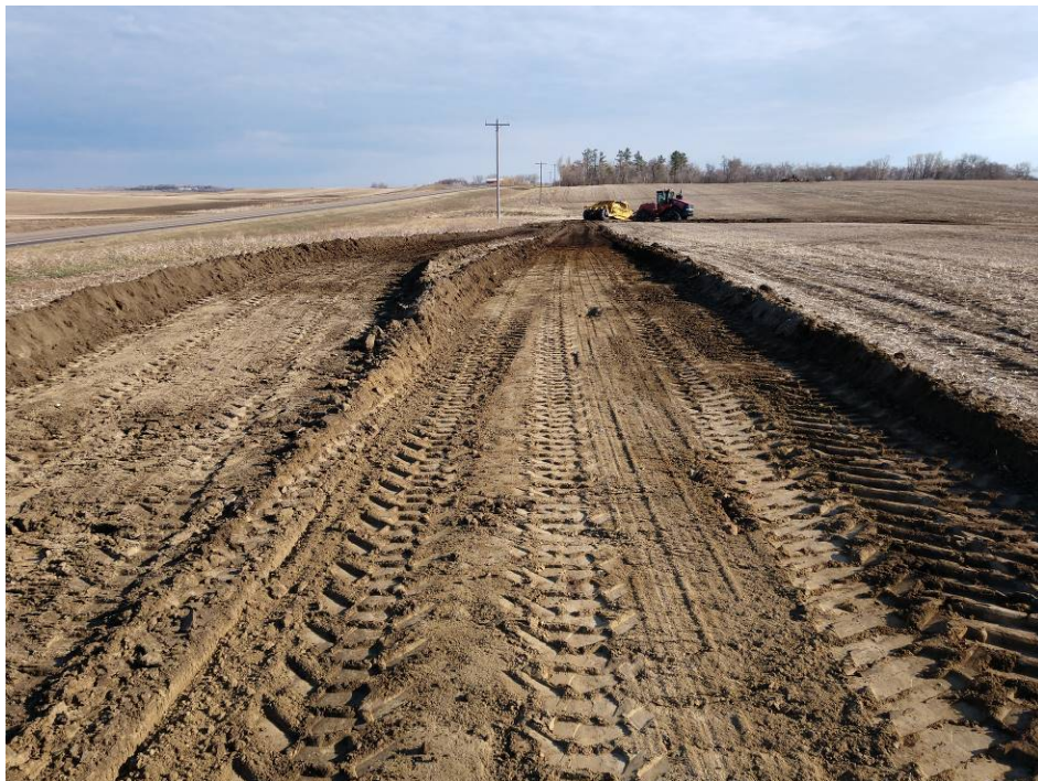
Figure 6. Photo taken looking north along west side of lay down yard.
