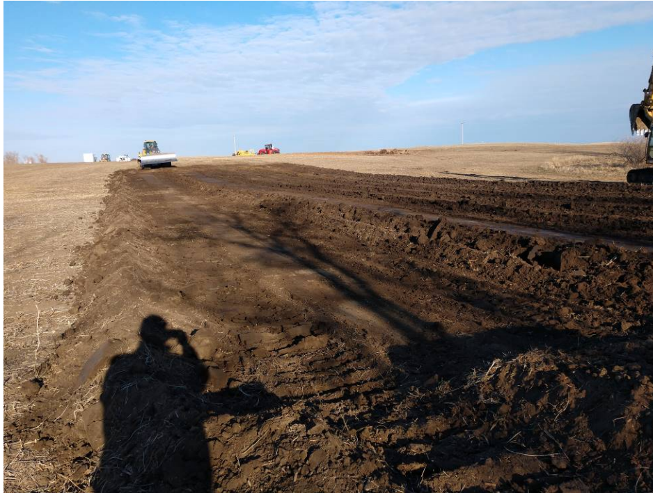
Figure 3. Topsoil stripping near southeast corner of laydown yard, looking northwest.
