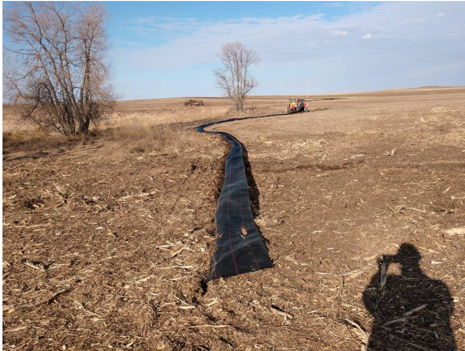
Figure 7. Installing silt fence along perimeter of wetland.
