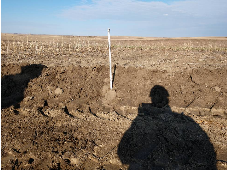
Figure 5. Photo showing depth of topsoil stripping. Topsoil is approximately 10" – 12" in low lying and level areas.
