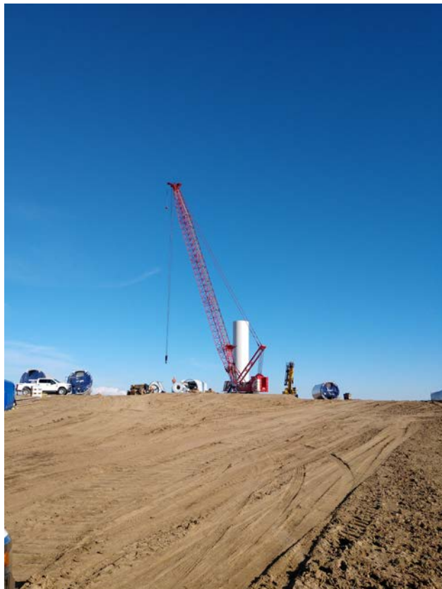
Photo 2. Photo of Turbine 13 pad taken facing east.
