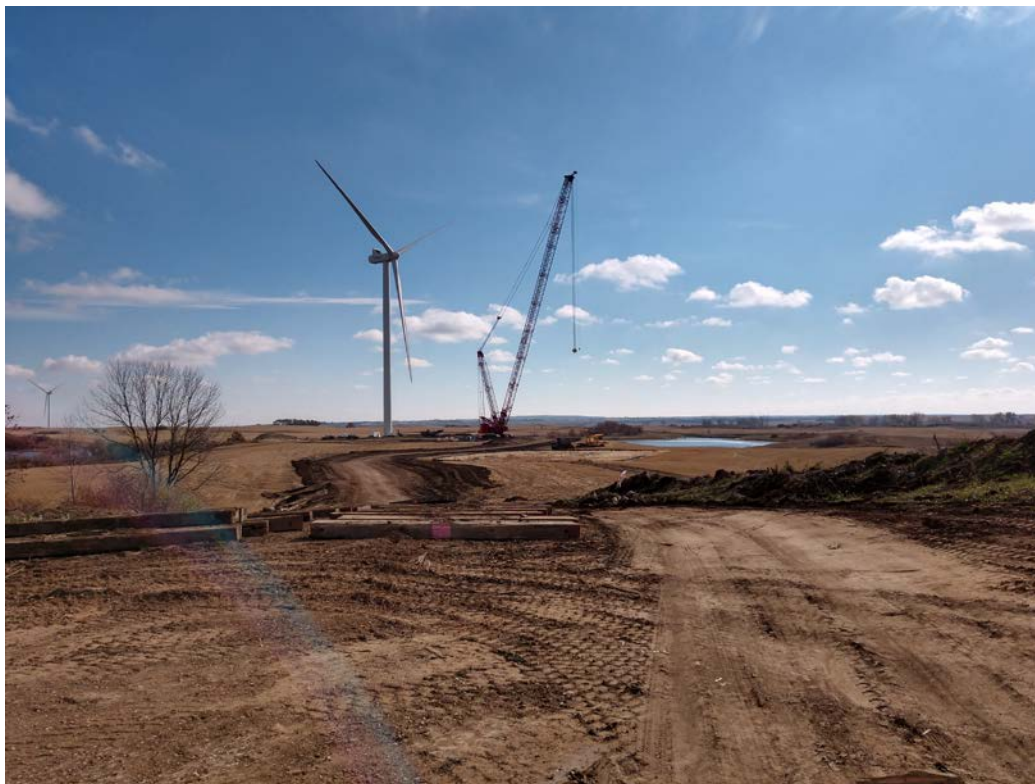
Photo 9. Photo of crane at Turbine 58 location. Photo taken facing east.
