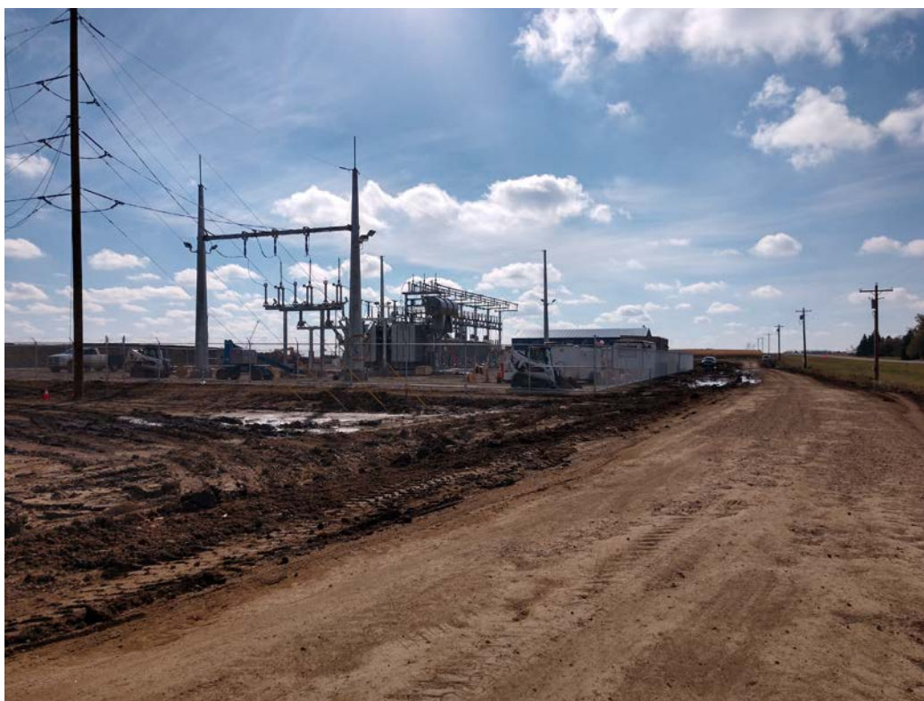
Photo 10. Photo of substation construction facing southeast.
