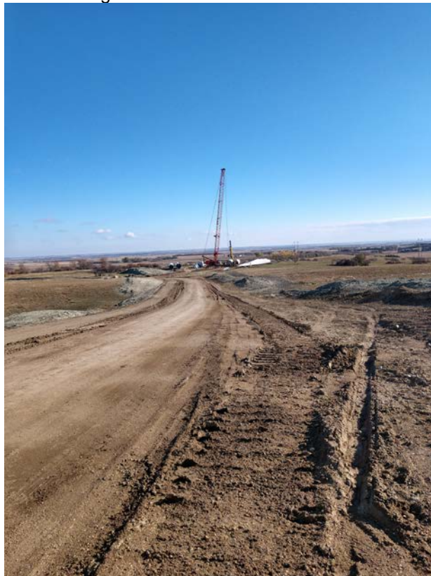
Photo 4. Photo of construction at Turbine 6 location facing northeast.
