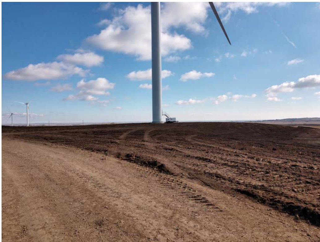
Photo 7. Taken facing east of earthwork around Turbine 42.
