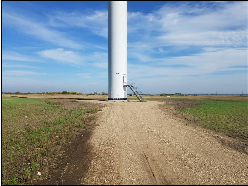
Photo 9. Photo of Turbine 64 facing North.
