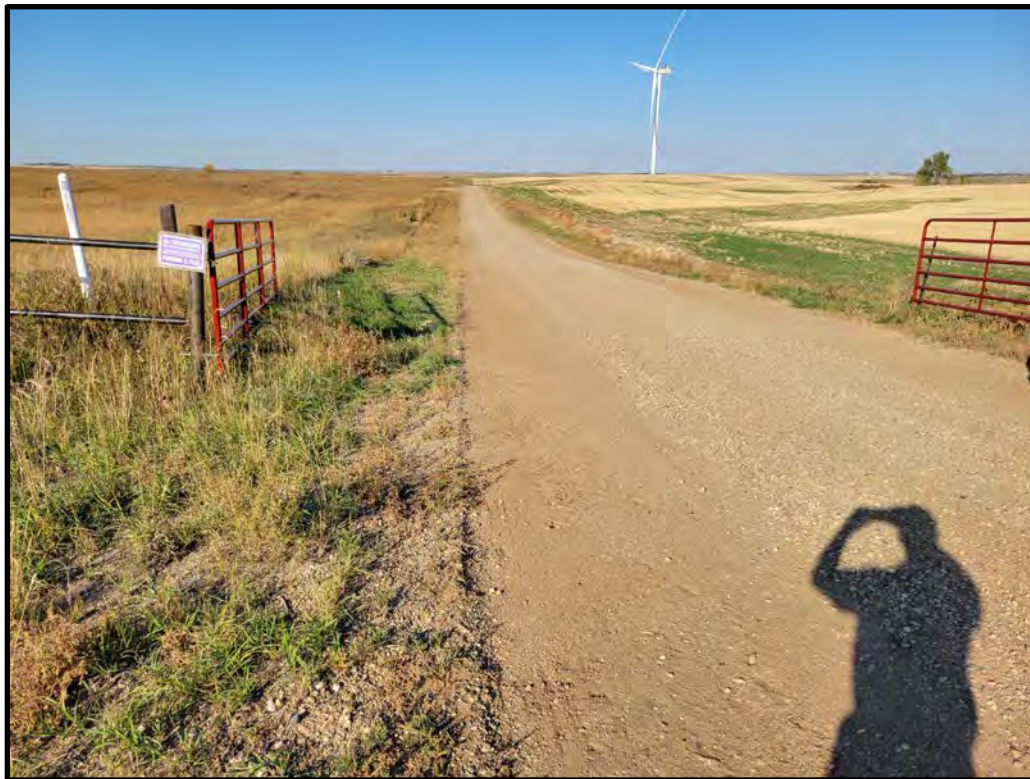
Photograph 1. View looking west along the access road to Turbine 31. Grass along the south side of the road was established.
