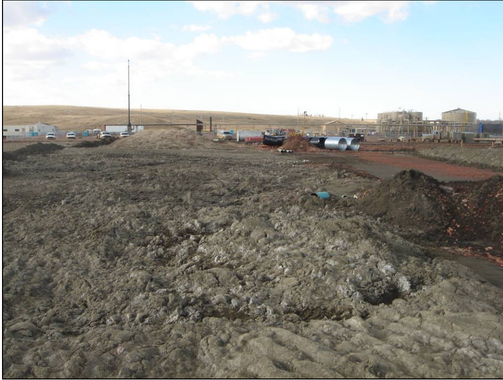
Figure 4. Project area overview depicting general topography at the eastern end of pipeline corridor, facing north.
