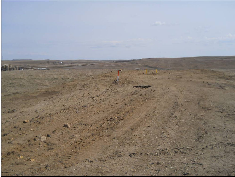
Figure 7. 32MZ782 site overview, facing north.
