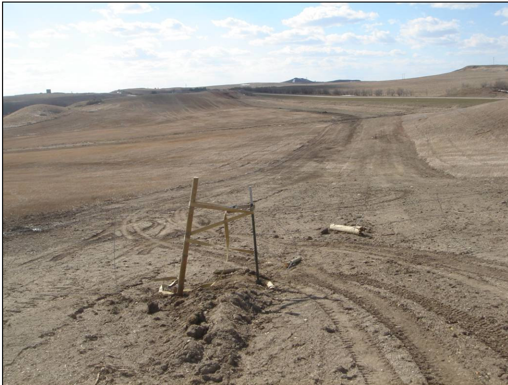
Figure 3. Project area overview depicting general topography on the western end of pipeline corridor, facing west.
