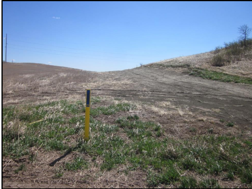
Photo 7. Direction: East. Pipeline route in the far northwest corner of the field from Photos 5 and 6, on the east side of 108 th Ave NW. Pipeline marker was in place in the east ditch. Note the bare, lighter colored soils on the hillslope which could be an indication of topsoil/subsoil mixing.
