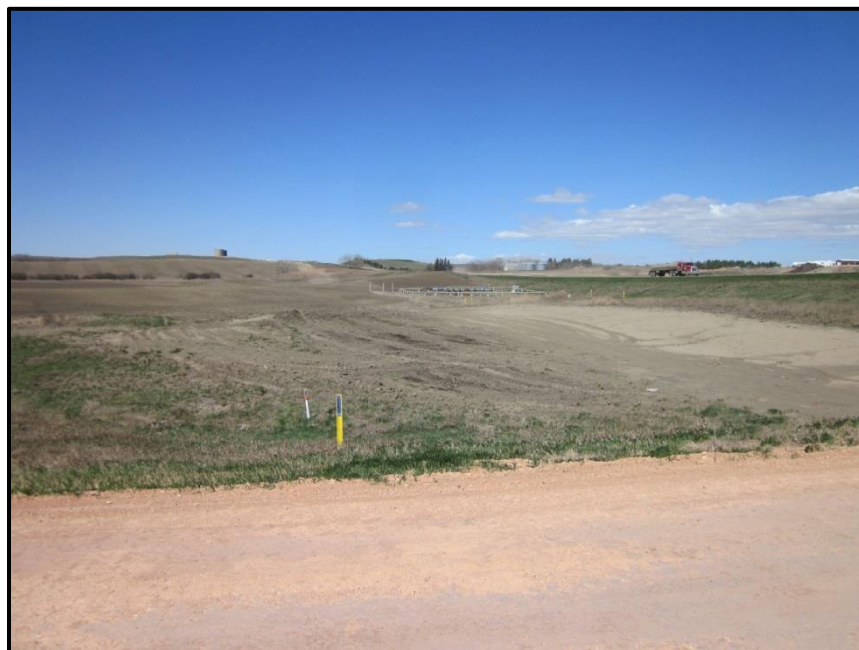
Photo 8. Direction: West. West ditch of 108 th Ave NW. The existing road had been bored underneath. Pipeline markers and cathodic protection system markers were in place. Note the light colored soils in the corner of the field, which could be an indication of topsoil/subsoil mixing. The core portion of the field had been planted for this year's crop, but this far corner had been excluded.
