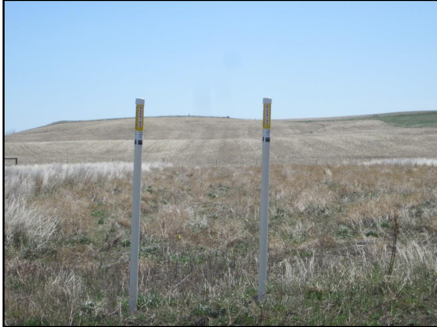
Photo 1. Direction: East. Pipeline markers on the east end of the pipeline which appeared to indicate an east-west routed portion of the pipeline, parallel to the south edge of the CDP facility. This route did not correspond to the submitted as-built drawings for the Project, which denoted that the pipeline was routed north-south in this area, but it could have also been the route of another pipeline. The field appeared to have been disturbed in the recent past (note difference in coloration), but was reclaimed properly and revegetation growth was good.
