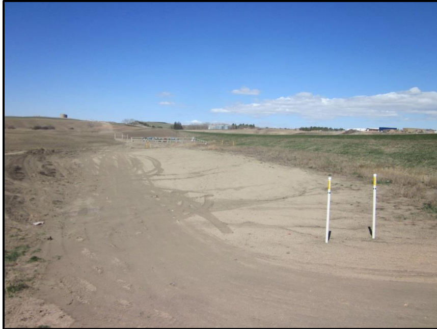
Photo 9. Direction: West. Markers were for an existing buried power line perpendicular to the pipeline route. Note the disturbed soils on the left of the photo where there were deep ruts (not visible) in the upper portion of a drainage, presumably due to heavy equipment, which needs repair. Otherwise reclamation was complete and soils were stabilized.
