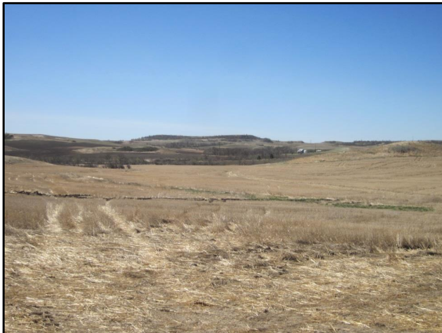
Photo 6. Direction: Southwest. View across field in the NW \frac{1}{4} of the NW \frac{1}{4} of Section 19. The pipeline route turned straight west across the remainder of the field. Reclamation appeared complete and the soils were stabilized.
